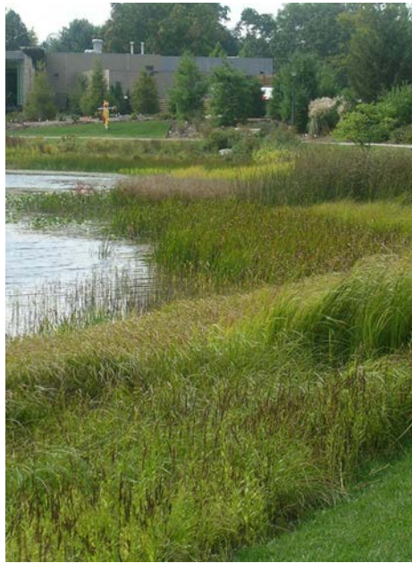
Flood storage area
