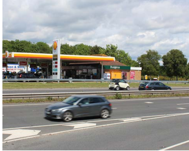
Photograph G - Petrol Station
