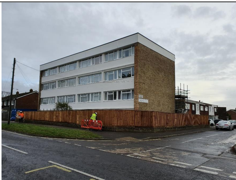
Photo 2 - Front/Side Elevation showing boundary fencing following works.
