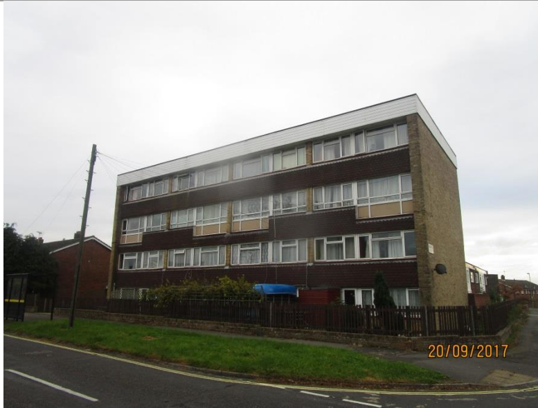
Photo 1 - Front Elevation showing boundary fencing prior to works
