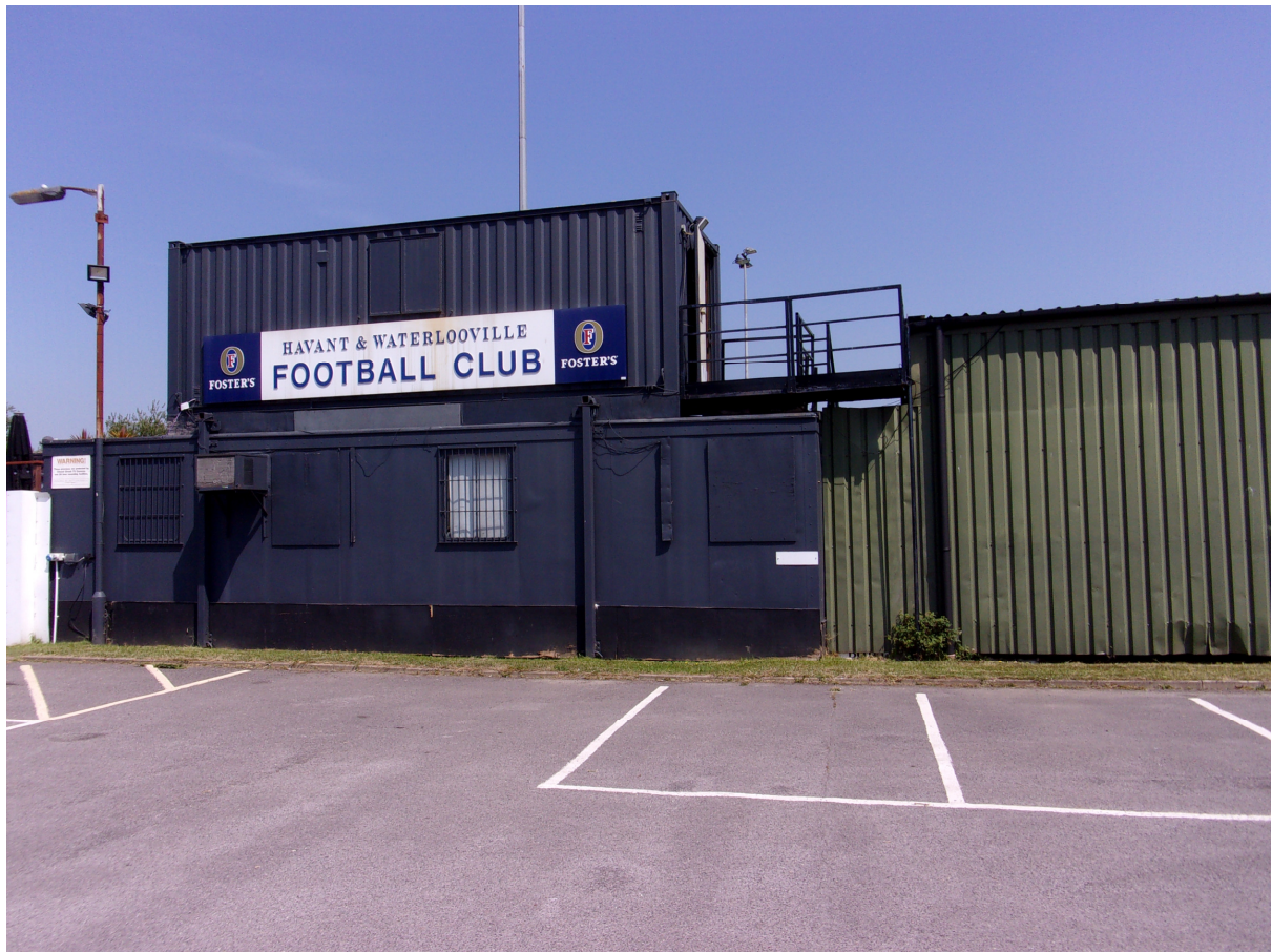
View of existing Portacabins to be removed
