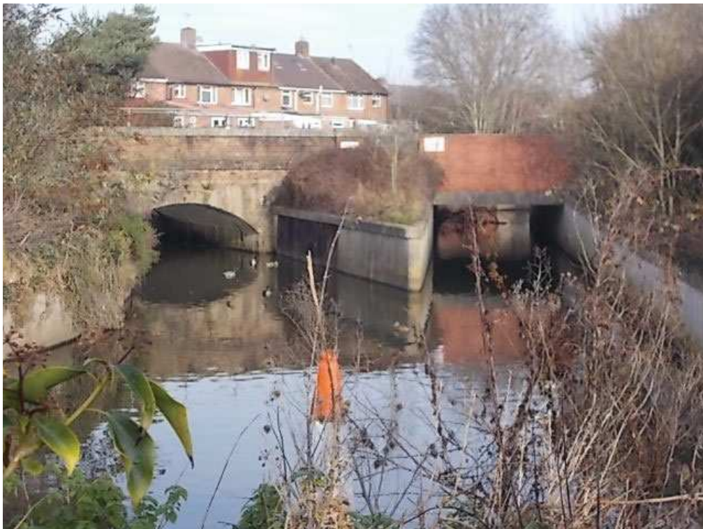
View looking north towards railway bridge spans ( site behind wall on RHS)
