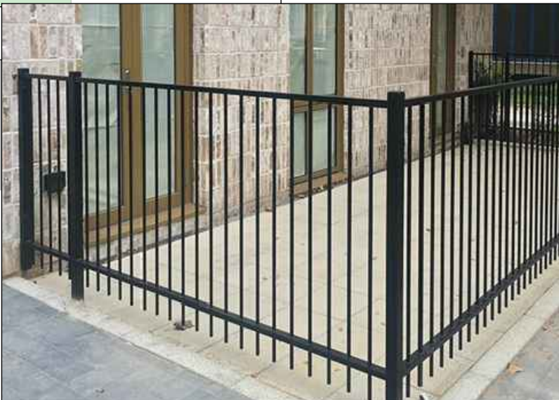
Black metal railings
