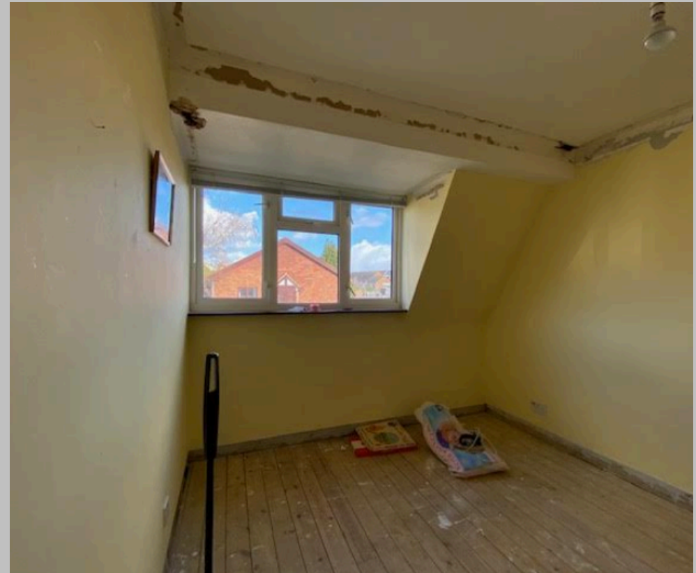
second floor bedroom interior view east facing (rear)
