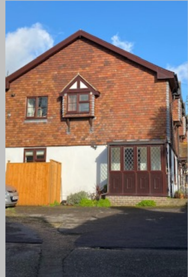
adjacent properties to rear
