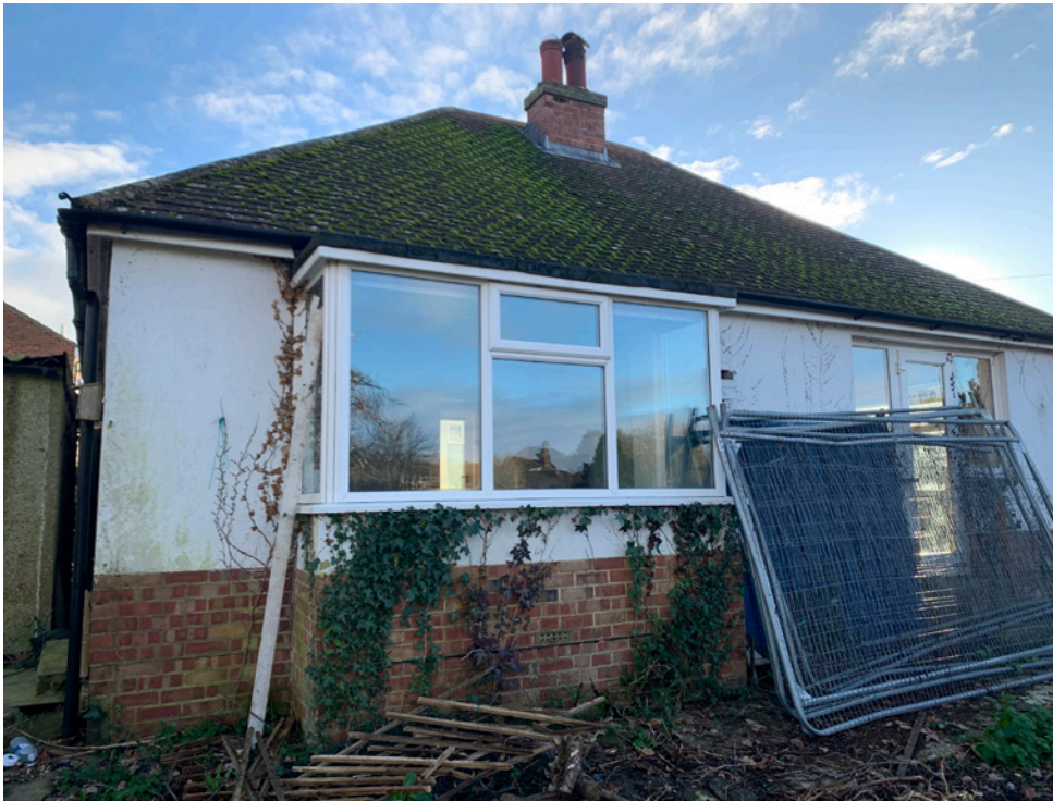
1A St James Road - West elevation
