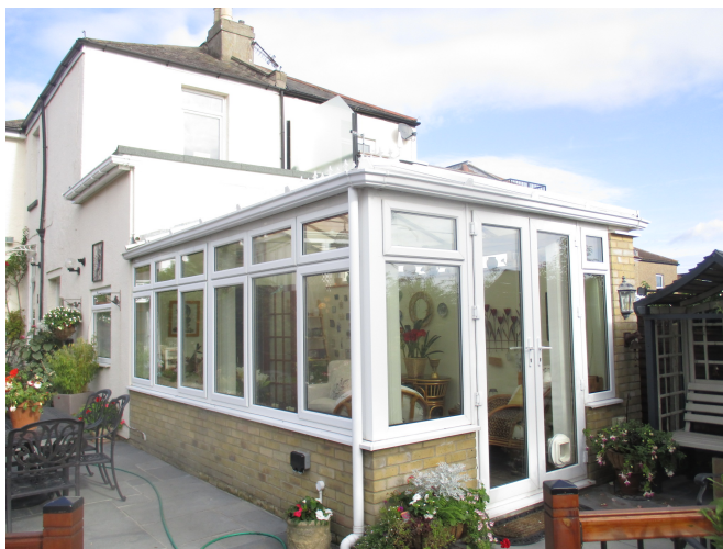
Fig 2– Existing rear of the property with flat roof extension. The view also shows the neighbouring properties balcony with privacy screen.
