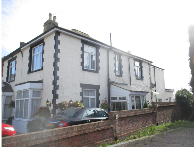
Fig 1 – Existing property viewed from Bedhampton Hill Road.
