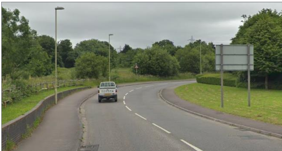
Image 16: Shared Footway / Cycleway along Lakesmere Road
