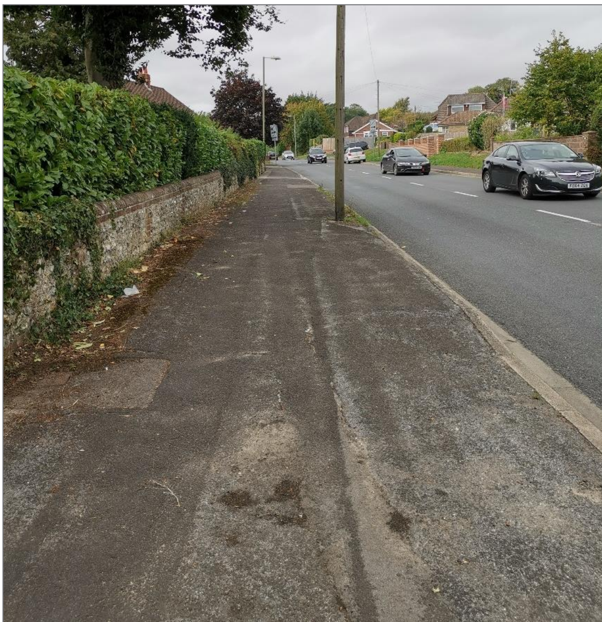
Image 3: Footways along Lovedean Lane
