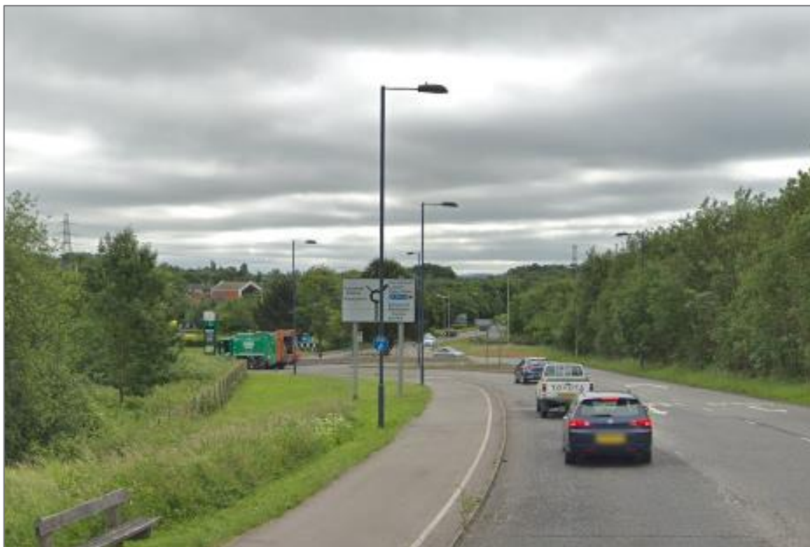
Image 15: Shared Footway / Cycleway along Dell Piece Way
