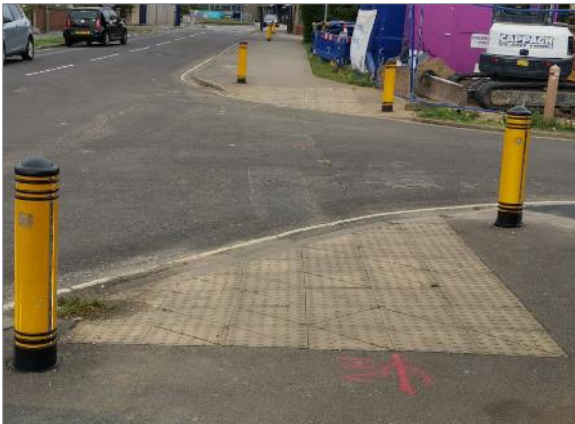
Image 13: Dropped kerb crossings with tactile paving on Barton Cross
