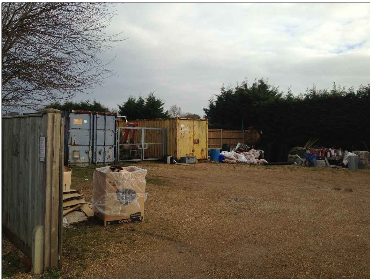
Plate 6: North-East corner of builders yard
