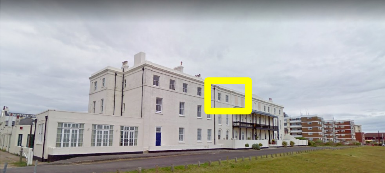
South aspect of The Royal Apartments, indicating our two South facing windows:
