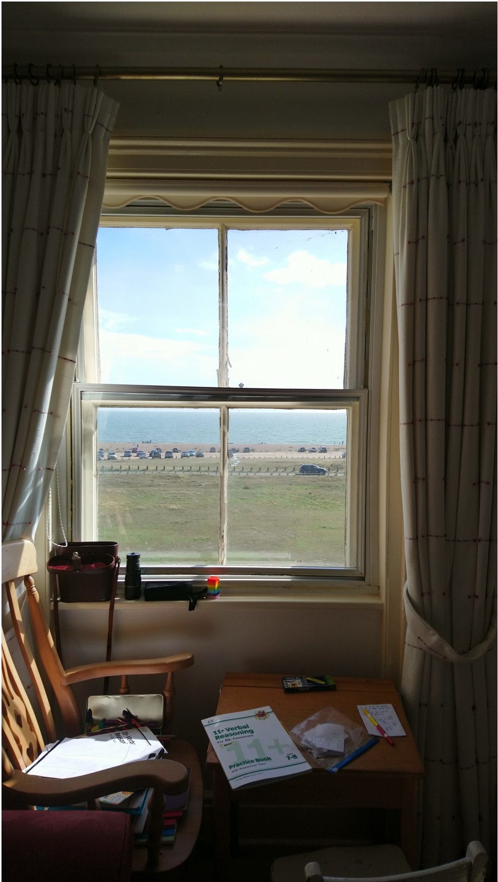
General view of current window style (modern internal secondary glazing to be removed):
