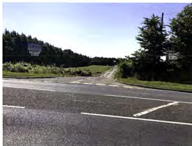
Photograph 2: Existing Site Access
