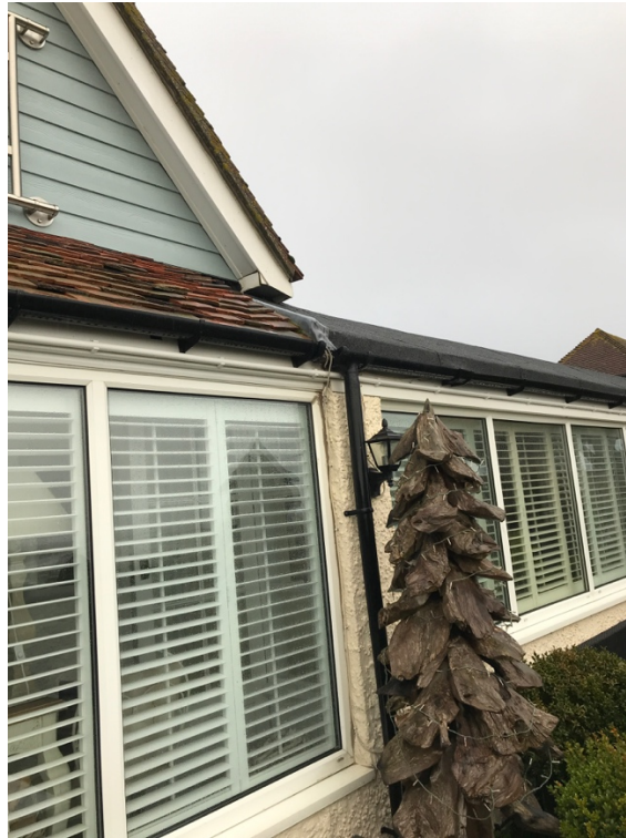
The tile and felt roof to be replaced with zinc roof with standing seams
