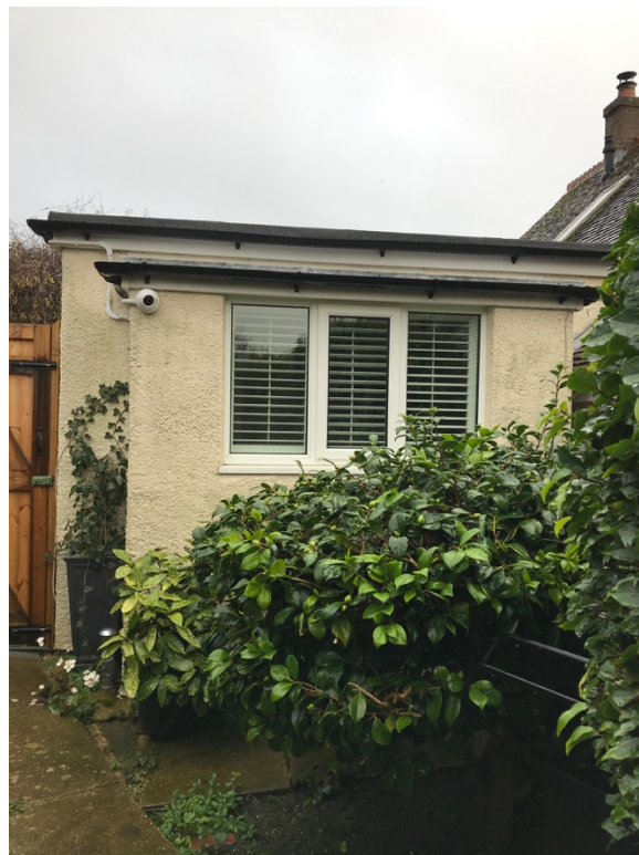
The existing flat roof extension on the east elevation (west view)
