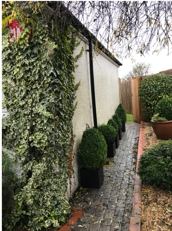
The existing single storey flat roof extension on the east elevation (east view)
