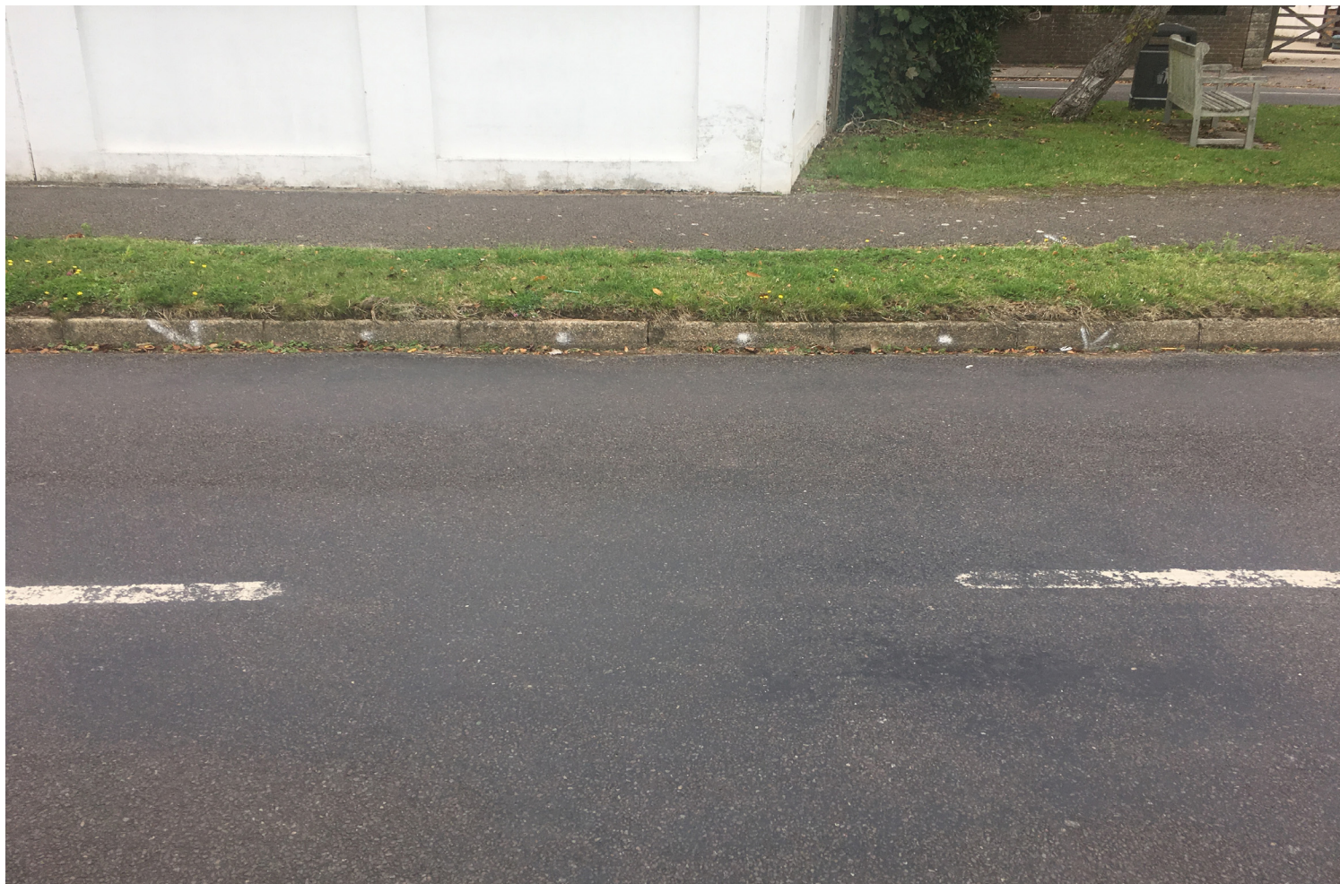
View 4 - Approved drop kerb location
