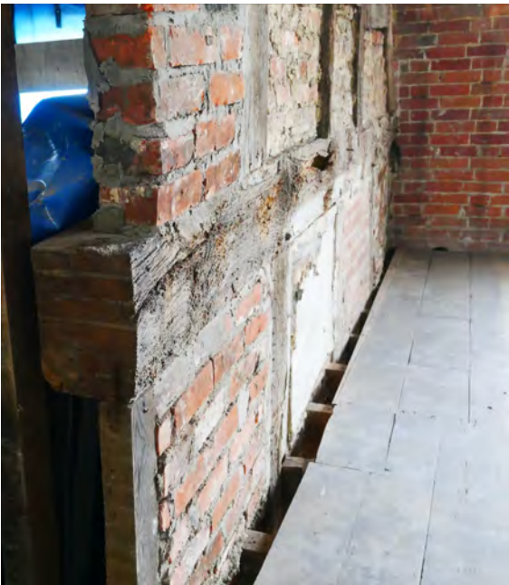
71. Truncated end wallplate for new opening. Infill panels would have had wattle and daub but have been replaced with brick.
