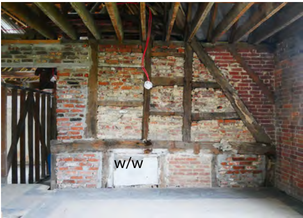
69. View of southern end bay
