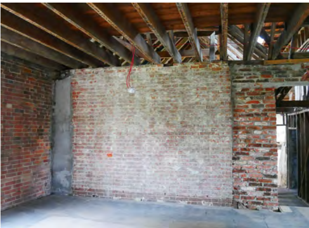
70. FF6 north wall, built after FF5. The rafters are of the Victorian period and a late construction.
