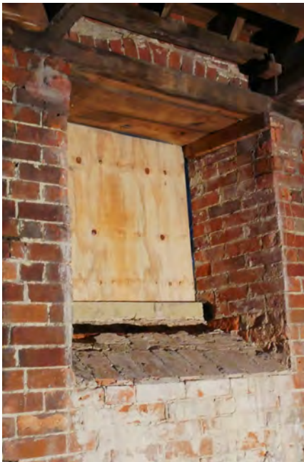
74. Small window to south gable of Victorian cross-wing.
