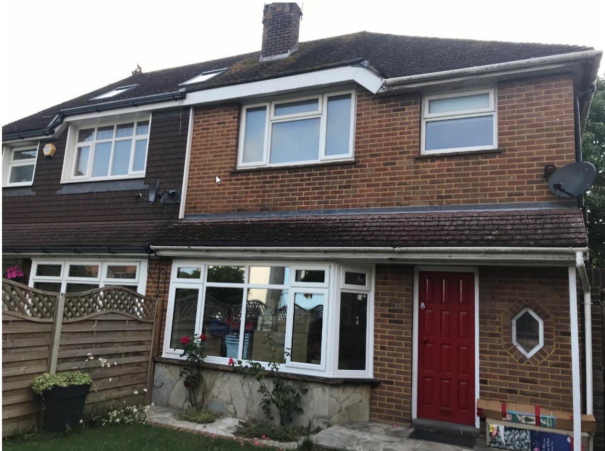
Front of the dwelling East Elevation
