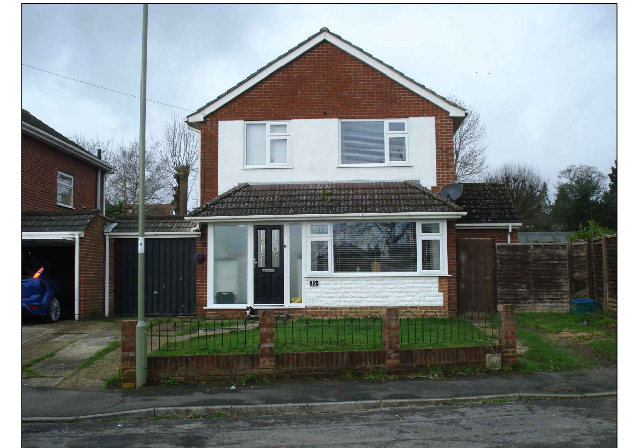
PHOTOGRAPH OF FRONT ELEVATION
