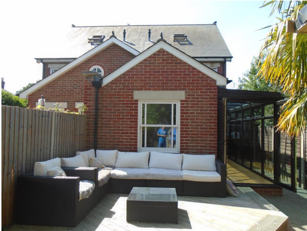
Figure 2. The rear of the dwelling.
