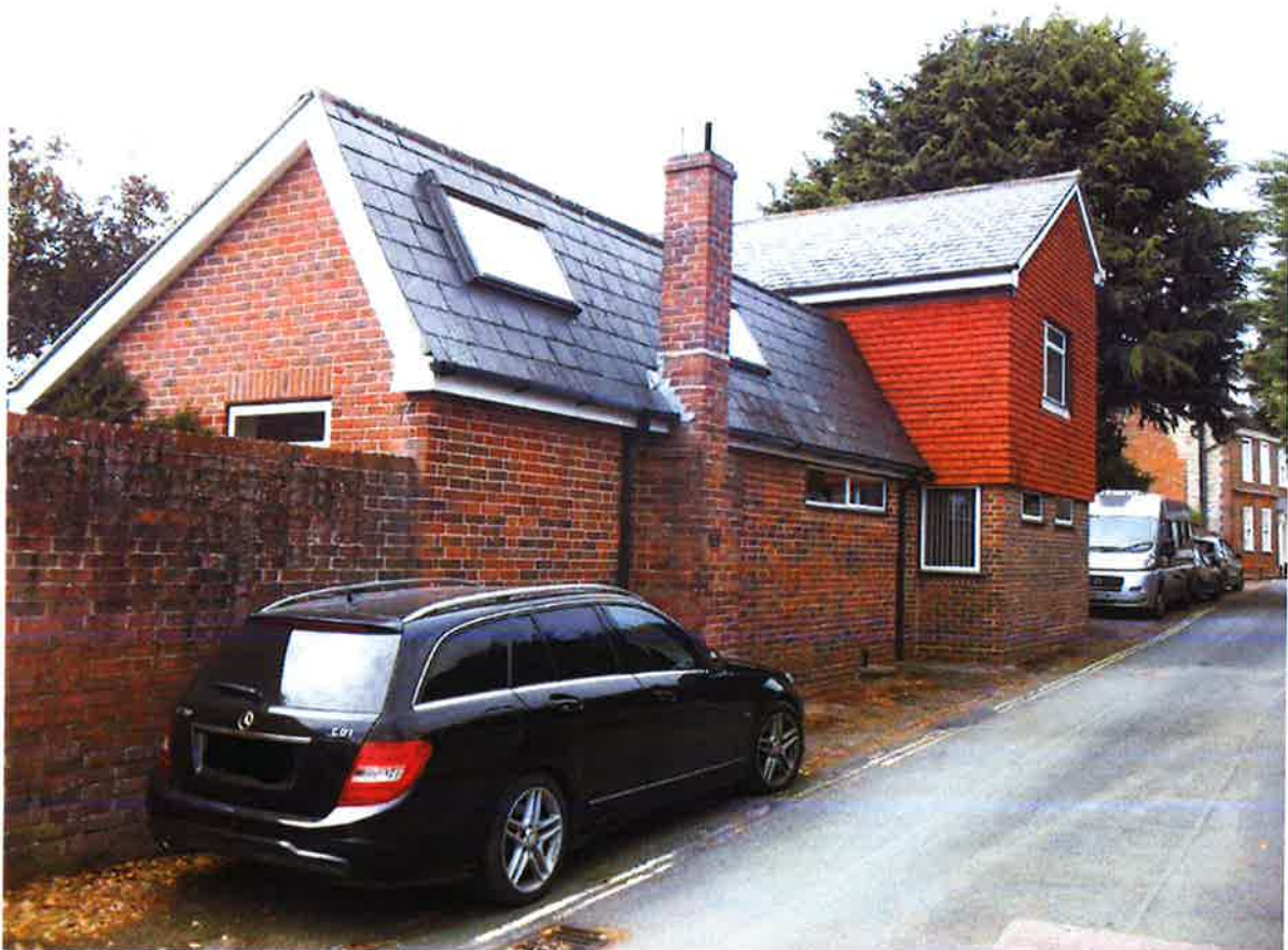
Photo 03 – Little Saxted, Tower Street Adjacent to the application site.
