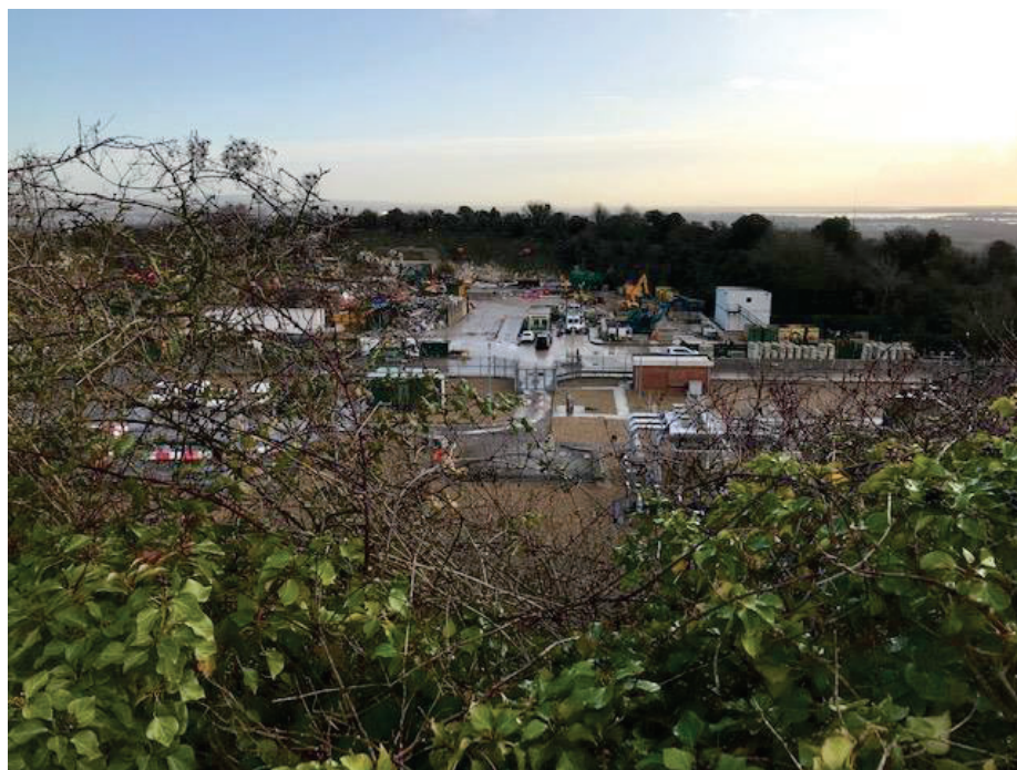
Plate 4: View east from the scheduled covered-way between Fort Purbrook and Farlington Redoubt towards the gas distribution facility.
