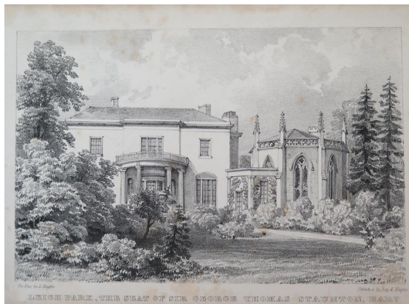
Staunton House and the Gothic Library 1832
