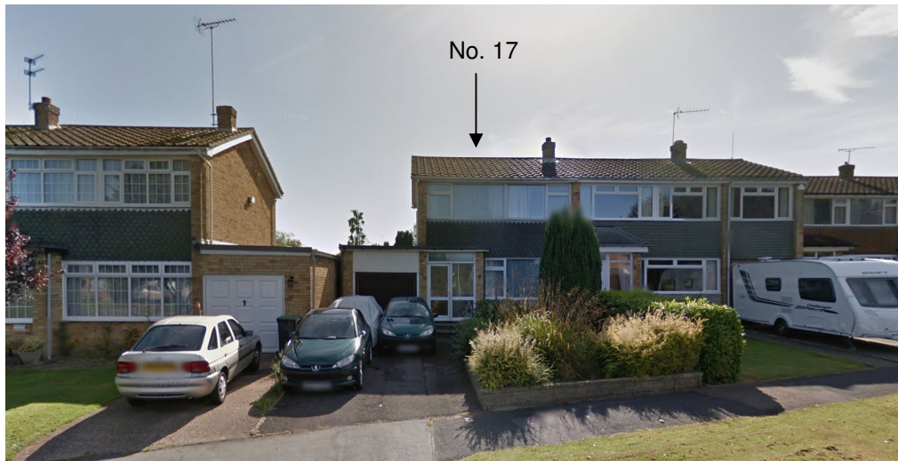
Fig 1 – View of the property from the road, with relationship to neighbouring properties (street scene).
