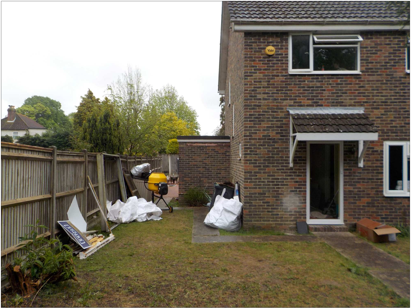
Front of 216 Havant Road, Hayling Island - showing proposed location of garage and parking
