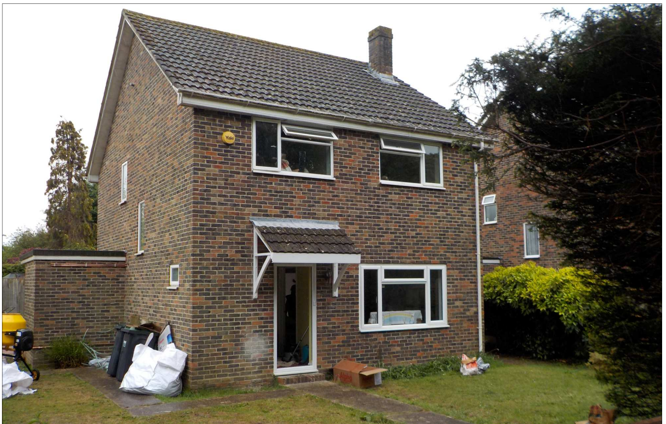
Front of 216 Havant Road, Hayling Island
