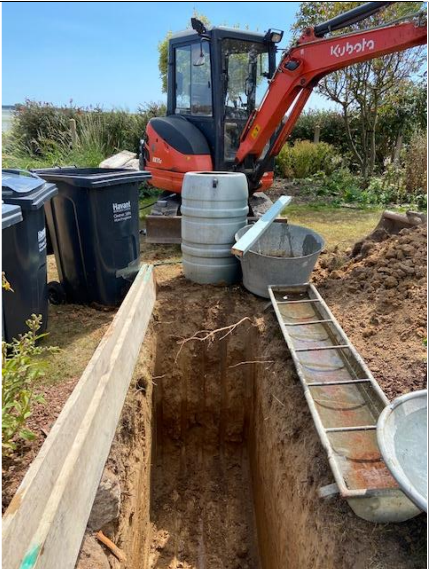
PLATE 2 – Soakaway SA2 – av. 1.85m long x 0.8m wide by 1.5m deep located in the front garden. As the length sloped from 2.2m at the top to 1.5m at the base although the average is 1.85m the average length at the water level is 1.79m
