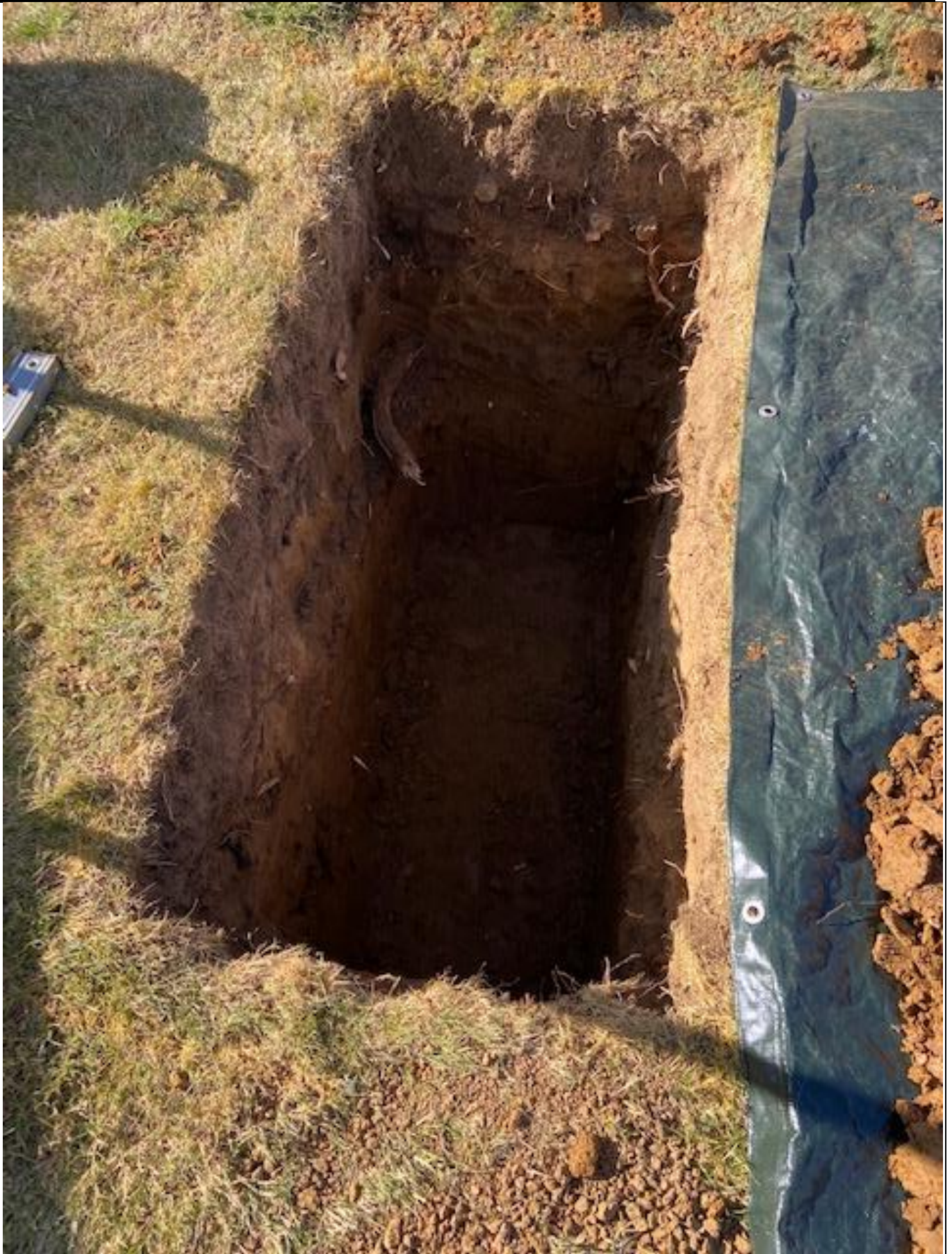
PLATE 1 – Soakaway SA1 – 1.5m long x 0.65m wide by 1.2m deep – hand dug in the rear garden
