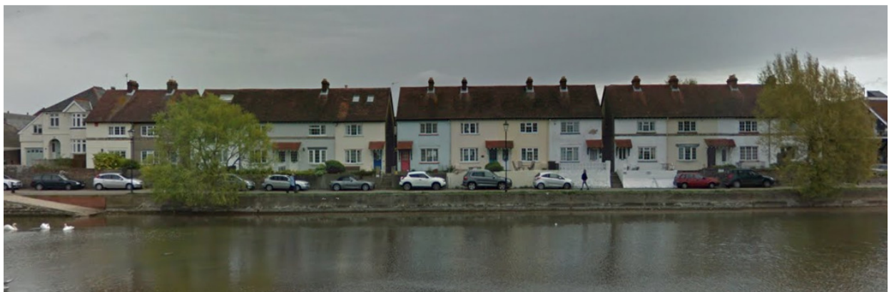
Figure 1, existing street scene along Bridgefoot Path. No.40 is the end of terrace – shown right hand side of the image, obscured by tree.
