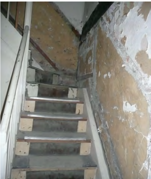
30. Ground to First Floor flight showing crossbeam, hidden rails.
