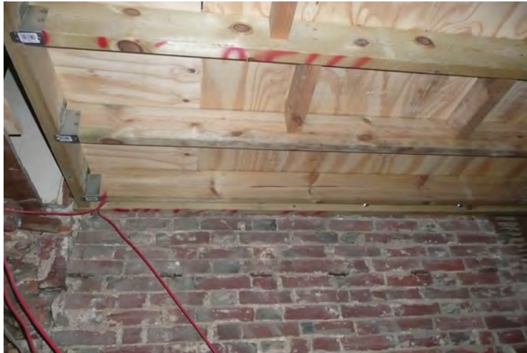
27. New floor inserted at higher level. Accepted that reversal would be harmful to historic fabric.
