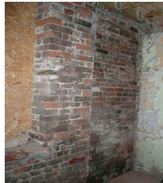
26. NW corner of G12. Previously partitioned off G11 as a utility room. Evidence of a former bay window clearly noted. Plaster had been applied direct to brickwork.
