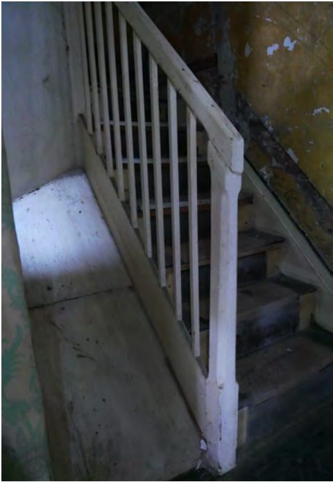
29. Newel Post, baluster and spindels of staircase, late Victorian.
