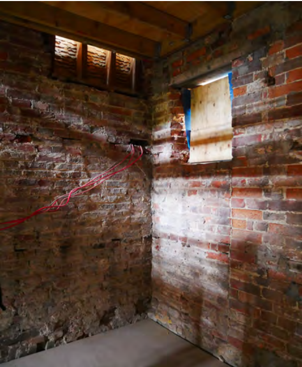
25. SW corner of G11, previously a wc. This was an extension to the north of the main entrance and west of central bay. The floor was been lowered in the past, revealing the cambered arch to the basement. The ceiling had been lower, cutting across the main windows. Now raised. Evidence of a former bay window can be said, a door at half landing height and a later small window.
