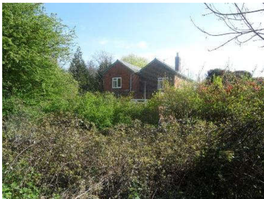
Fig 10. View of 32 Langstone Road (West Elevation) from the 'dismantled railway' public footpath to the rear.
