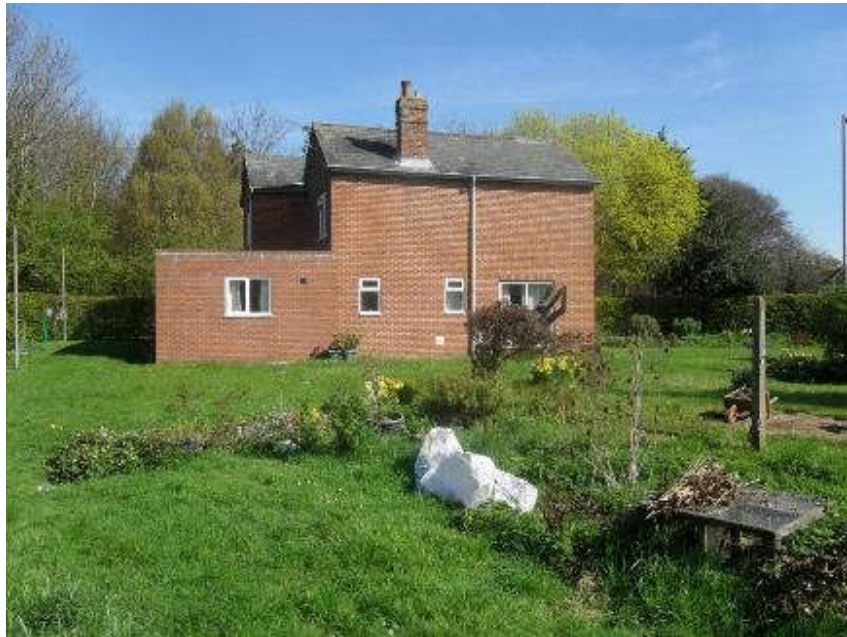
Fig 7. View of 32 Langstone Road (South Elevation).
