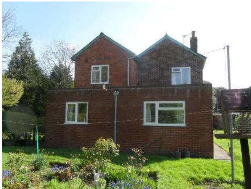
Fig 8. View of 32 Langstone Road (West Elevation).
