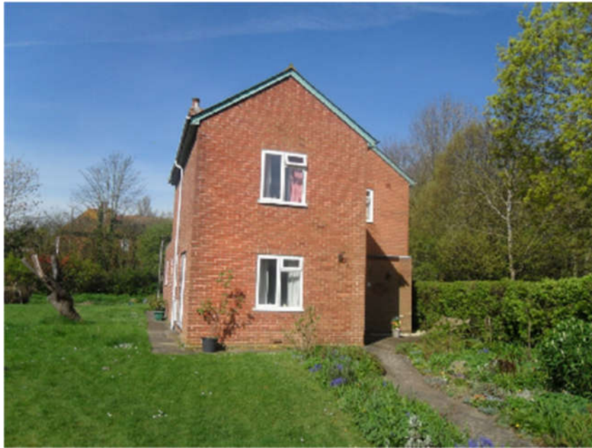
Fig 5. View of 32 Langstone Road (East Elevation).
