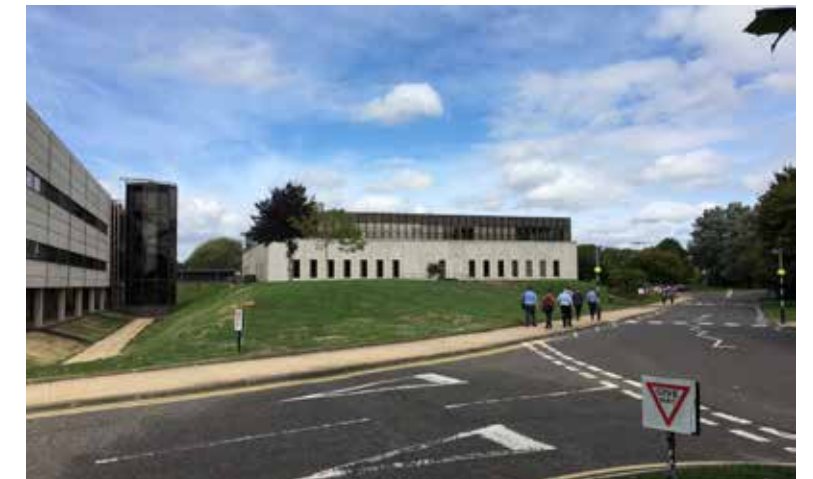
04 - Building 6000 east facade (left), Building 7000 and entry road visible centre right
