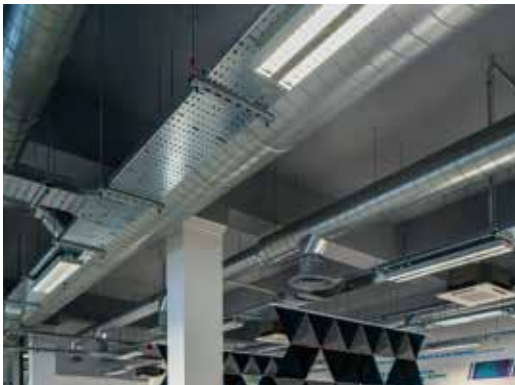
01 Exposed services soffit
