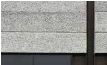
Existing concrete panels & channels
