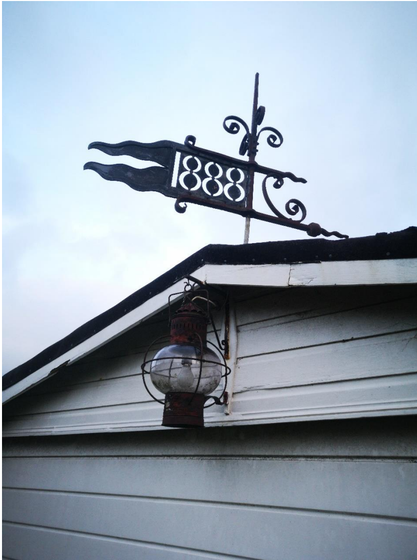
Existing wind vane and light which will be incorporated into the new garage build
