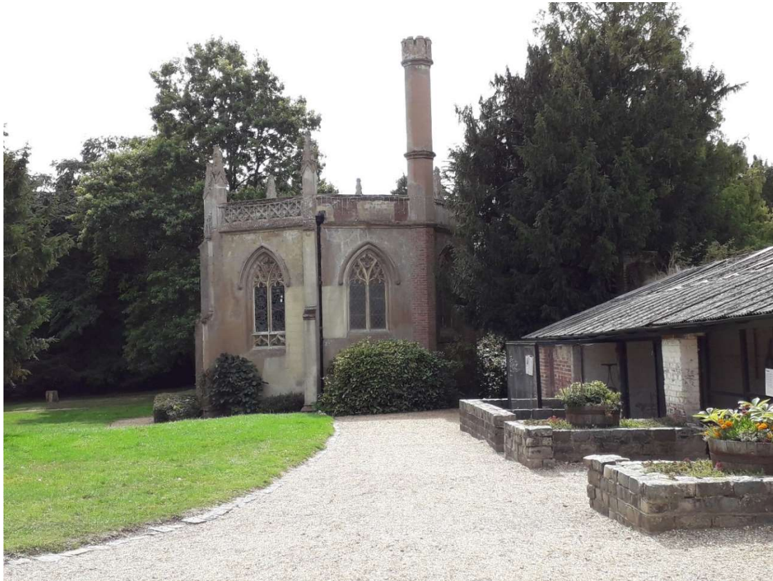
Fig 11. Current view of the Gothic Library from the Visitor Reception Building south entrance, with walled garden to right.
