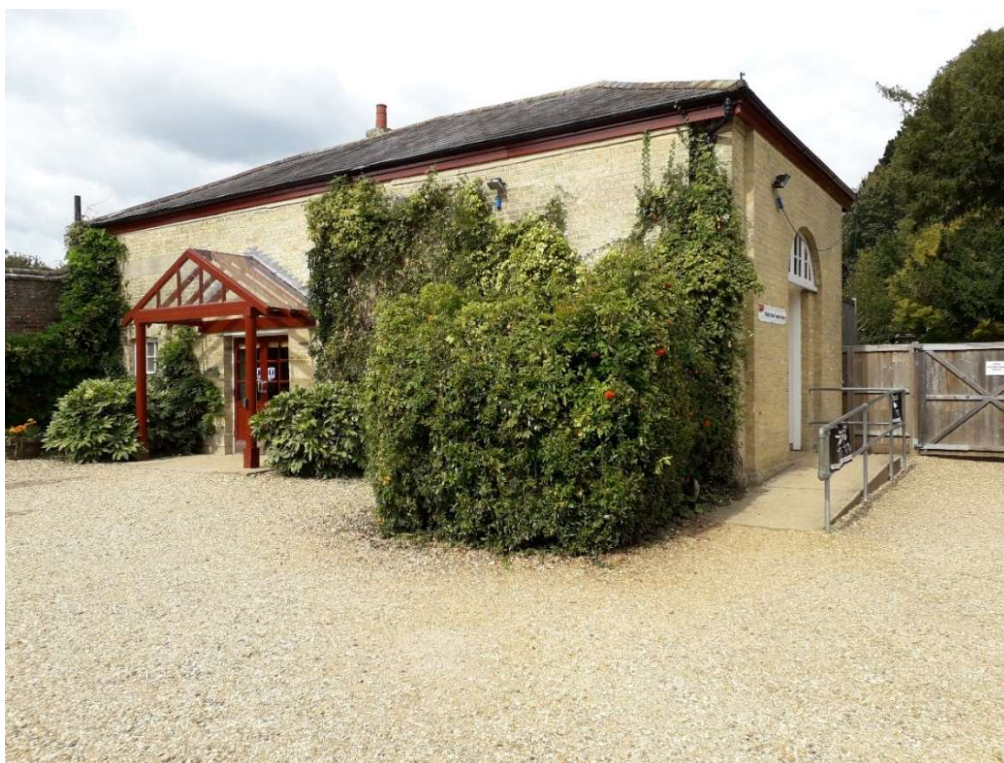
Fig 6. Current view of Visitor Reception Building from the south-east, showing building's south entrance (c 1992) and modern roof canopy (c 2013) and concrete ramp leading to wall opening on east elevation, where external hand-washing facility is situated (c 2013).
