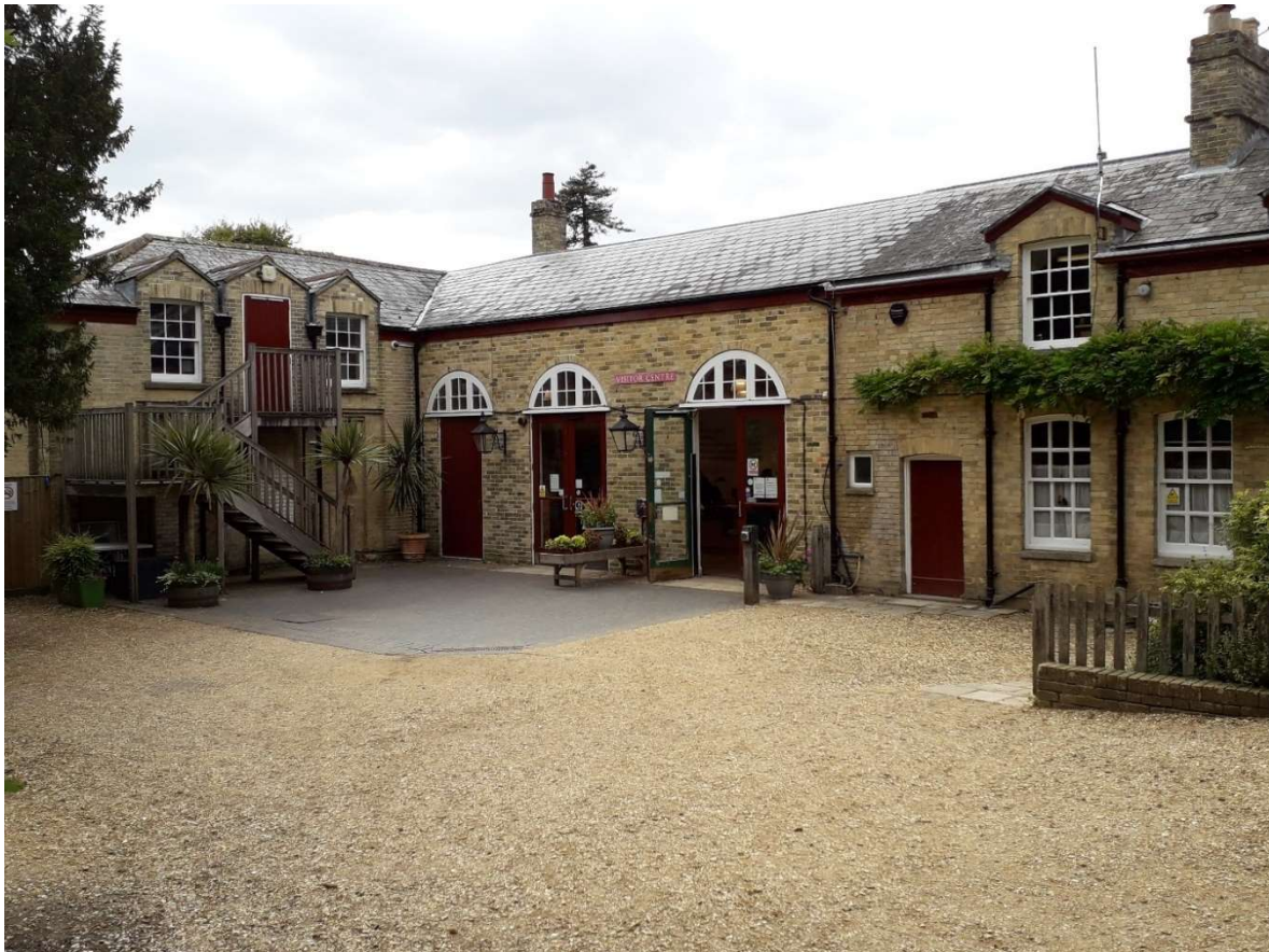
Fig 8. Current view of Visitor Reception Building with courtyard, viewed from north-east. The two-storey former Bothy is to the right (now Park offices) with new entrance doors and brickwork infilling in the centre, where the Coach House and Stable doors were located. Visitor toilets with Park offices above (accessed via external timber staircase) are accommodated in the south-east wing to the left.
