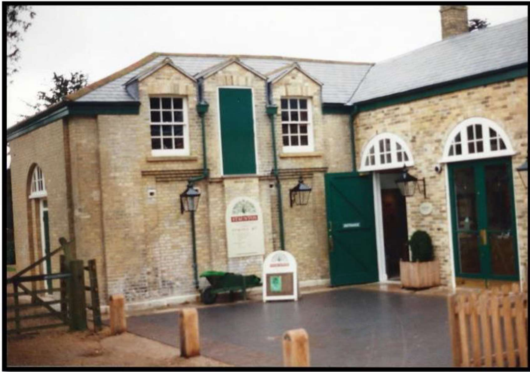
Fig 4. The courtyard viewed from north-east, after its conversion into the Visitor Reception Building in 1992. Note the demolished timber-framed staircase has not been replaced, new entrance doors to reception and retail area and external door to visitor toilets on east elevation.
