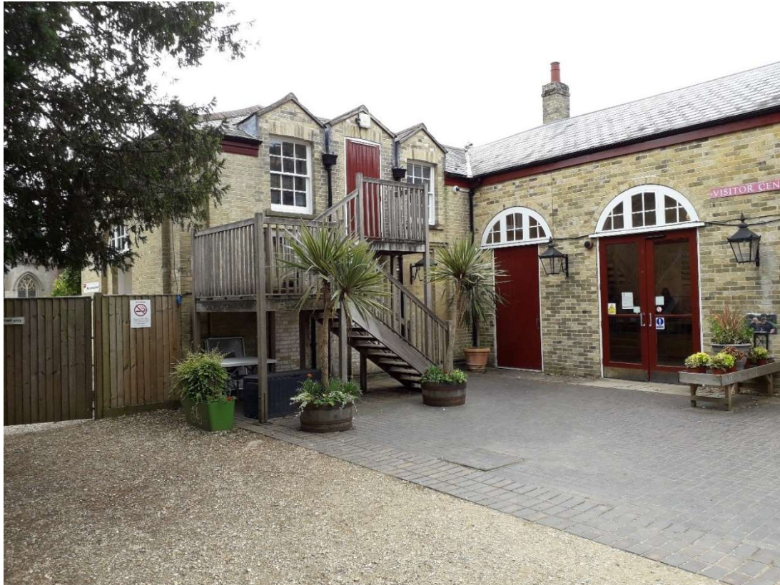
Fig 5. Current view of courtyard. Note installation of new external timber-framed staircase, circa 2013.
