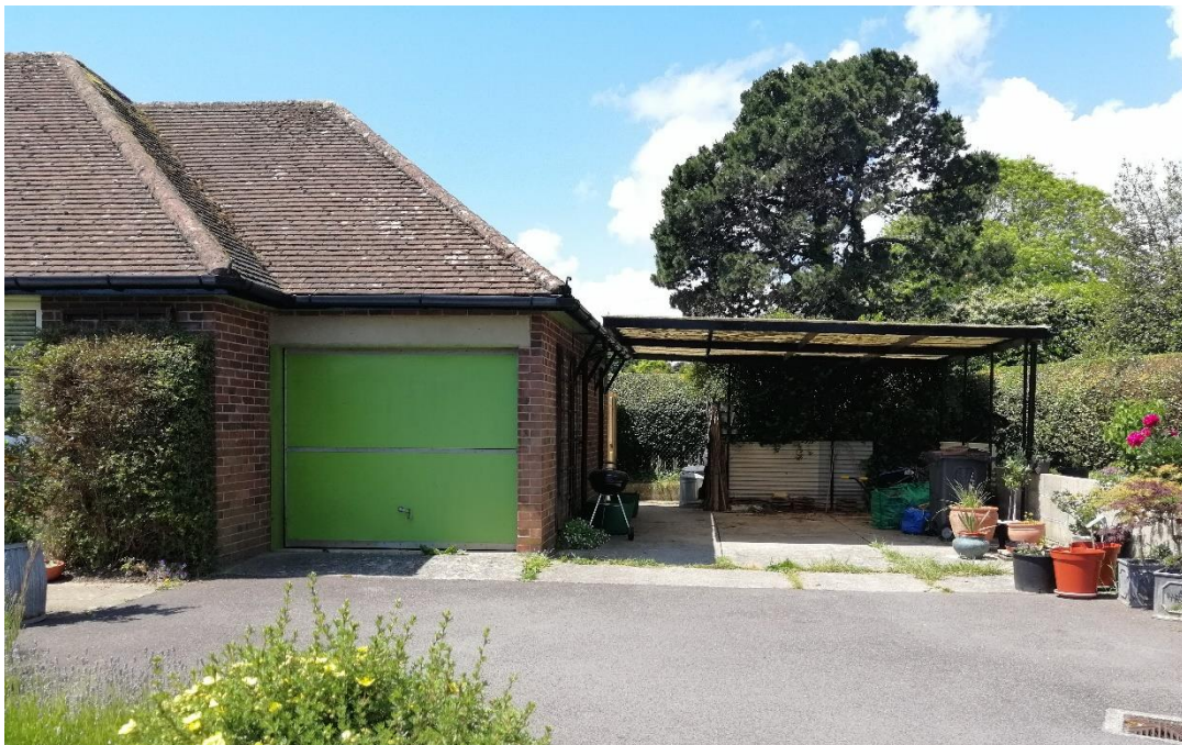
Figure 4: Garage and Pergola type roof structure.
