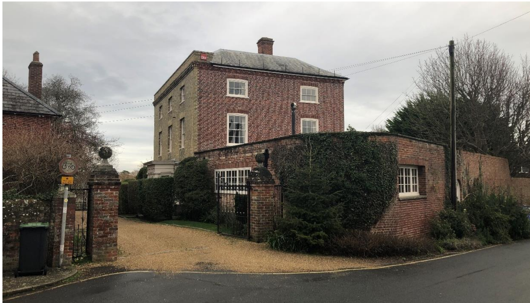
Photograph 1 – West (Side) Elevation
