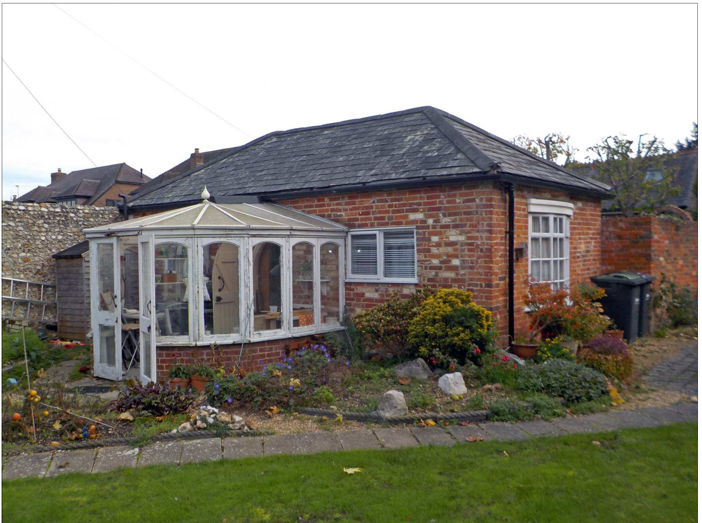
Workshop showing existing conservatory.
