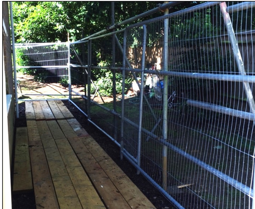
Scaffold board pedestrian ground protection
