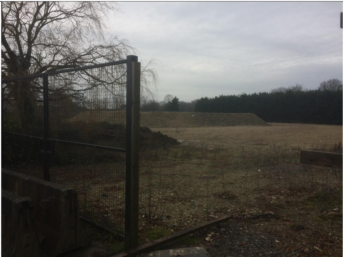
PLATE 2 – Site has been cleared with the concrete crushed and stockpiled in the centre
