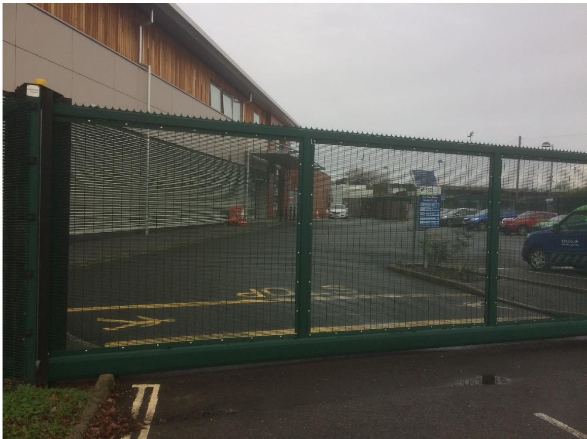
PLATE 6 – SSE offices and depot adjacent to south-eastern boundary
