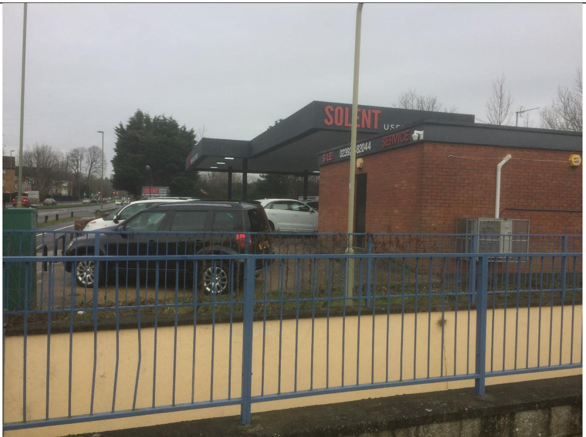
PLATE 4 – The used car dealership adjacent to the south-western site boundary
