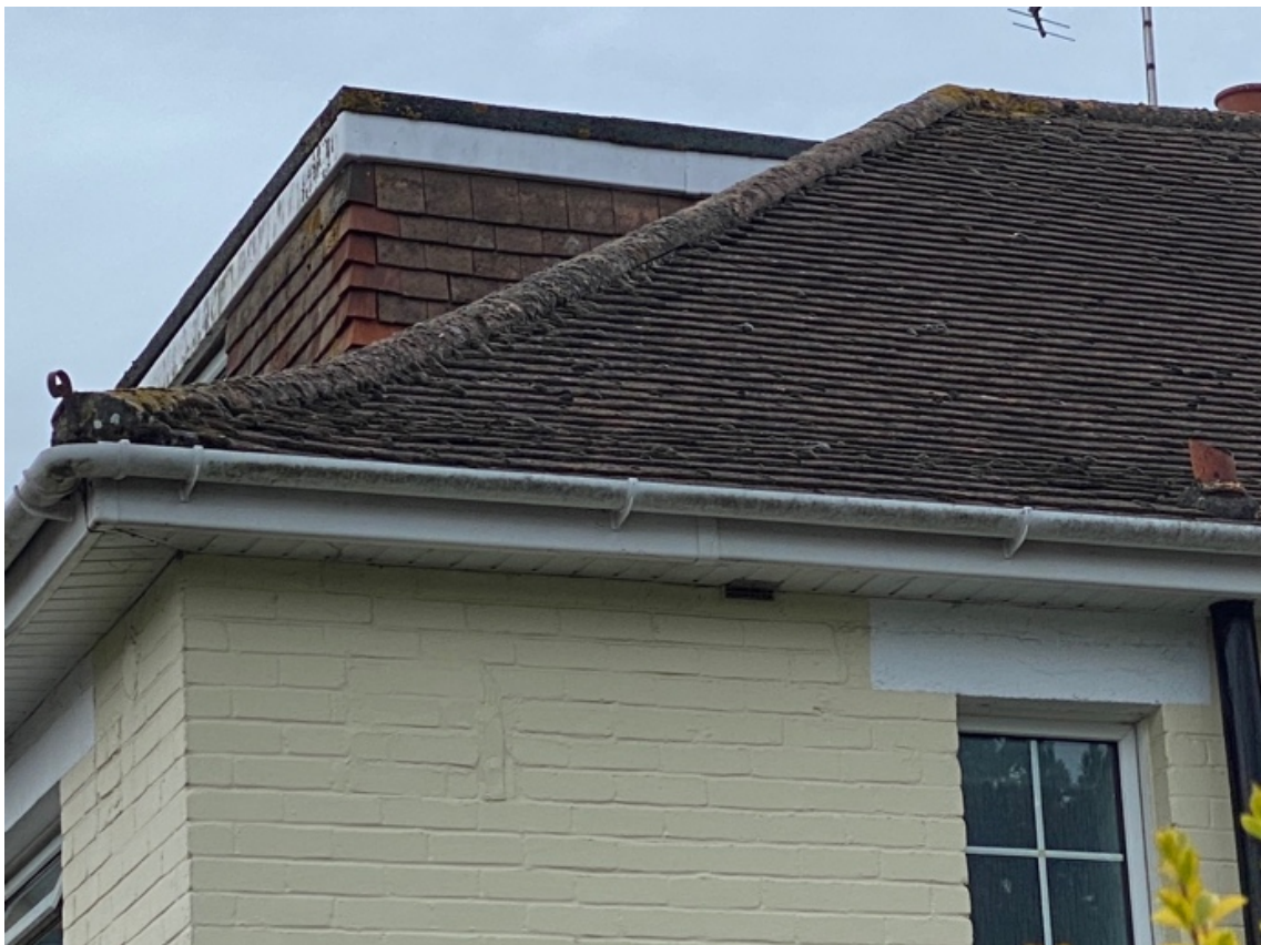
Existing roof tiles
