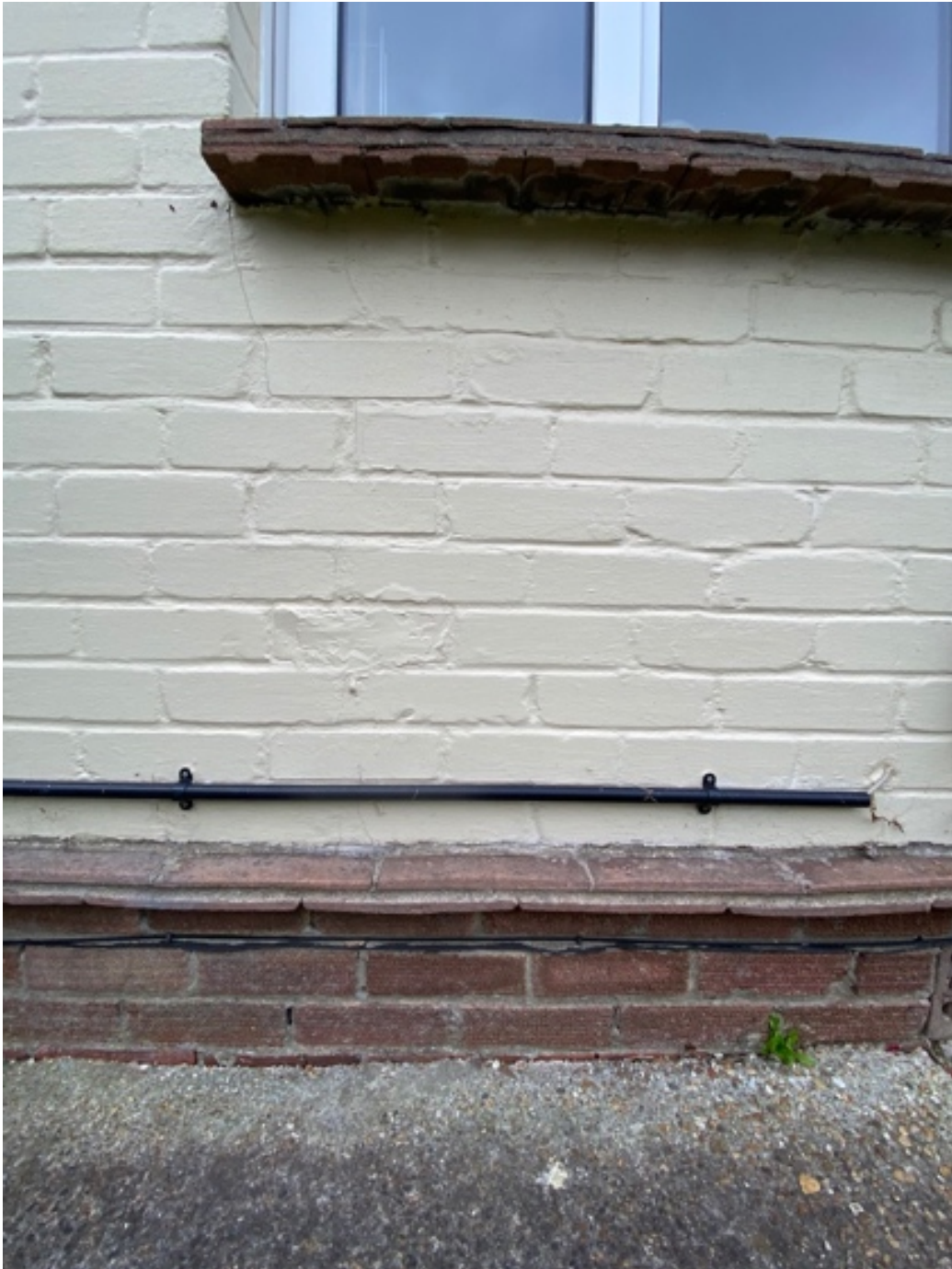
Existing wire cut bricks below dpc; clay roof tiles used as crease tiles; buttermilk colour painted brickwork above dpc and clay roof tiles used as window cills.
