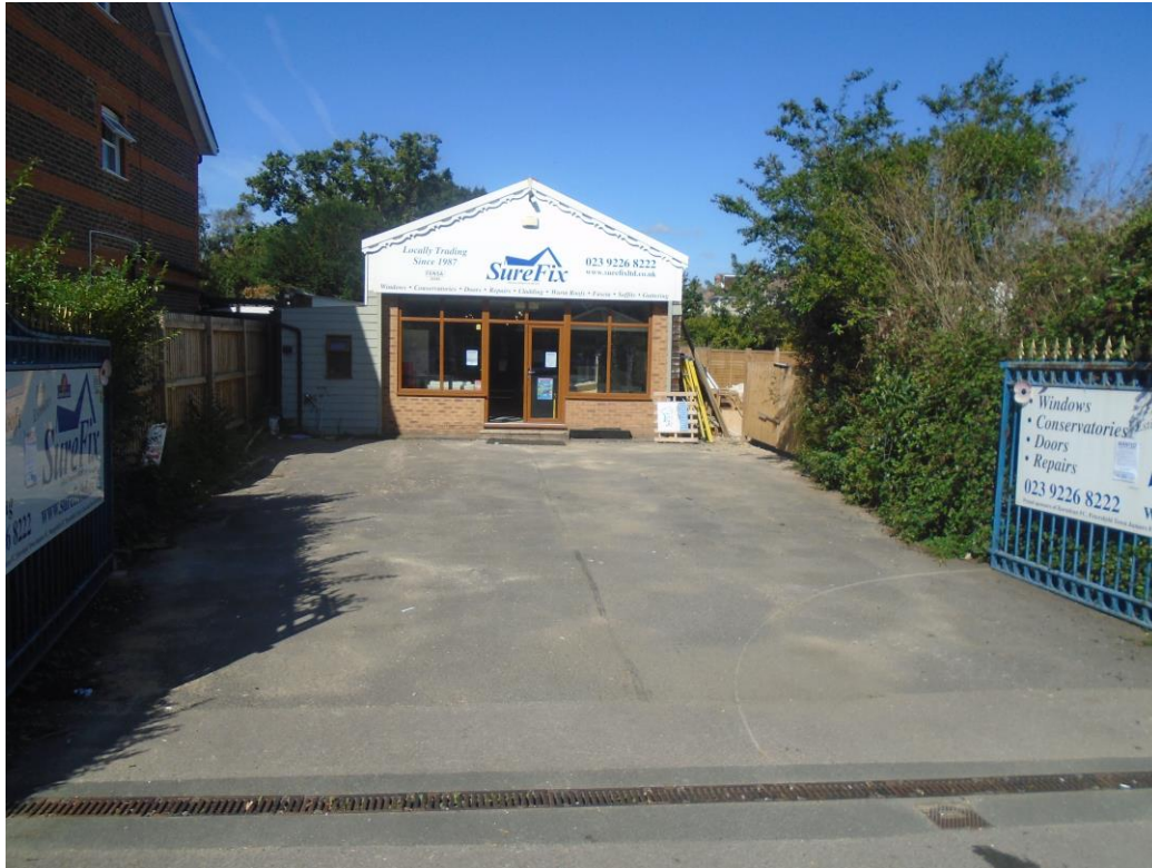
Figure 1. Frontage of appeal site to London Road
