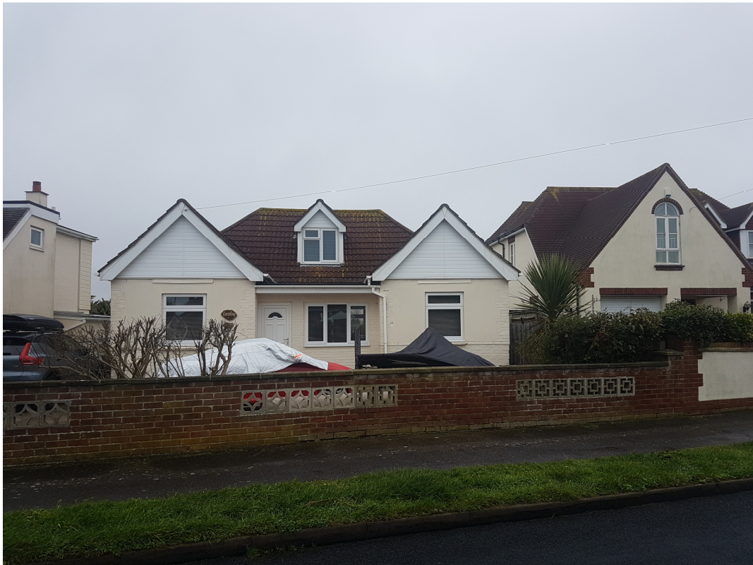
View of existing front.
