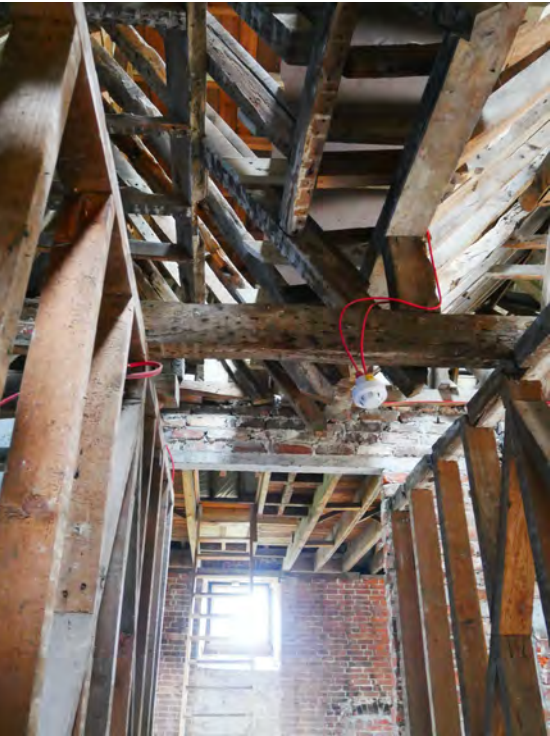
62. Valley between 2 roof above. Later partitions of each side.
