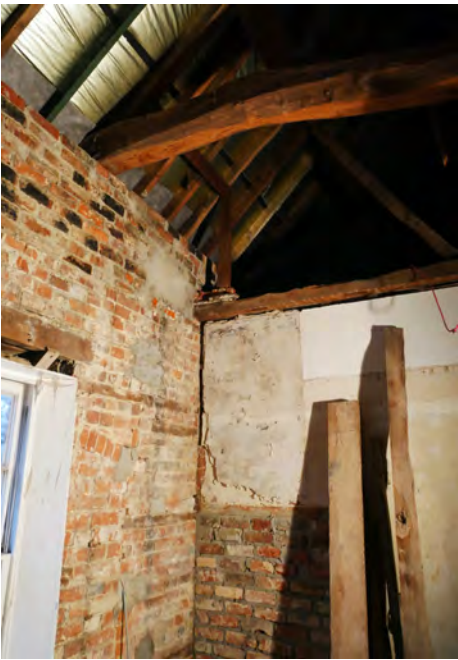
63. FF5 NW - Evidence of bay window. Note the outer west wall plate has been raised. The two walls do not match which indicates different builds.
