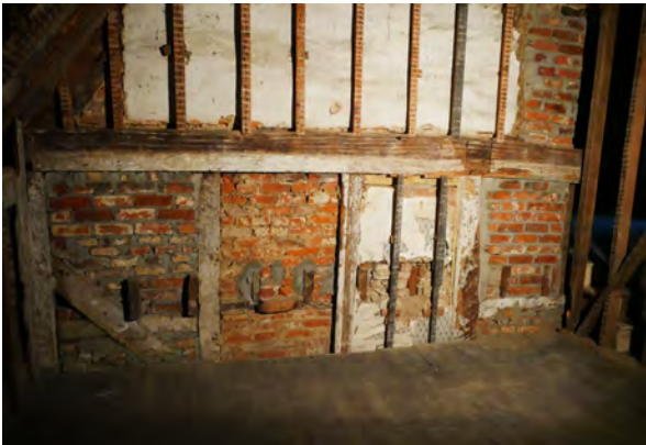
67. FF5 south. The joists of the 'new' floor can be clearly seen. End wall plate intact. Floor raised.
