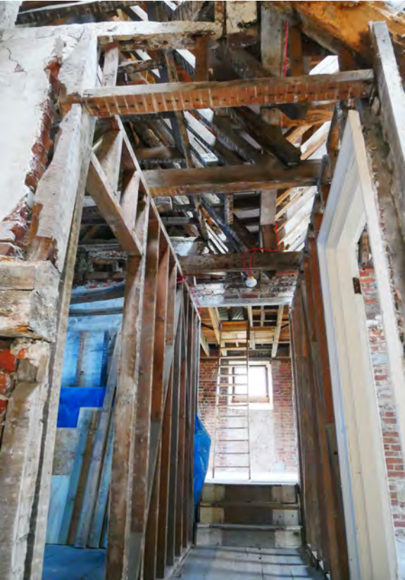
61. View from FF3 stair. This hall serves FF5, FF9 and leads to the later Victorian cross wing with attic above. Height floor to ceiling has been raised to 'fit' with the Victorian alterations.
