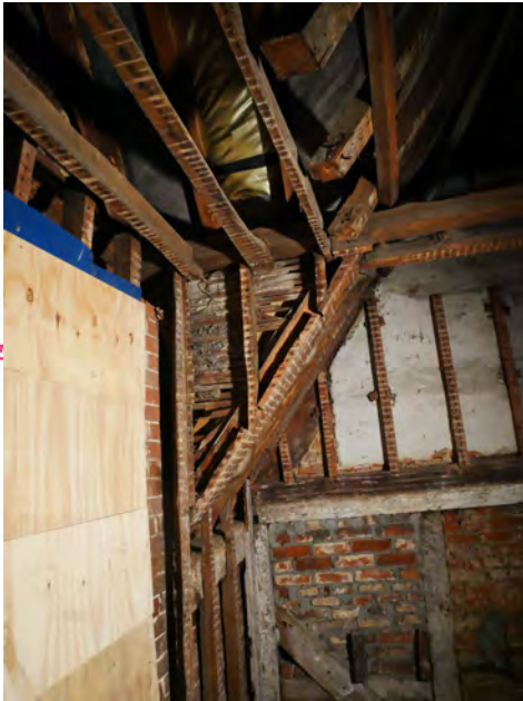
66. Raised wall. of a less substantial construction. Evidence of adaptations to roof incl. dormer introduced.
