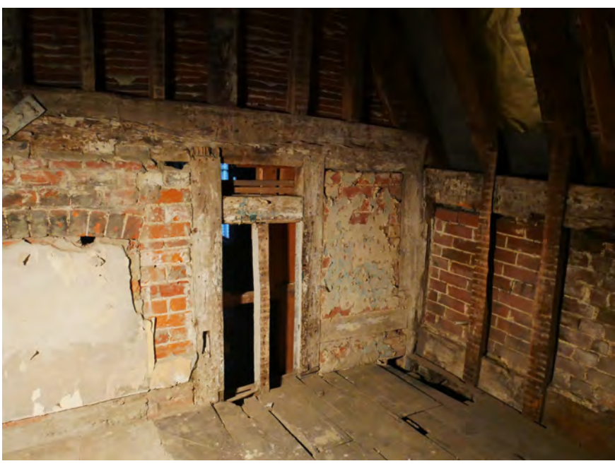
65. Nrtth & East inner walls -the south end chamber bay of the 3-bay post medieval house. The floor is notably raised. Cross beam and wall plate with jowl post to corner. Blocked up fire-place. The ceiling height had also been raised. This was covered over.
