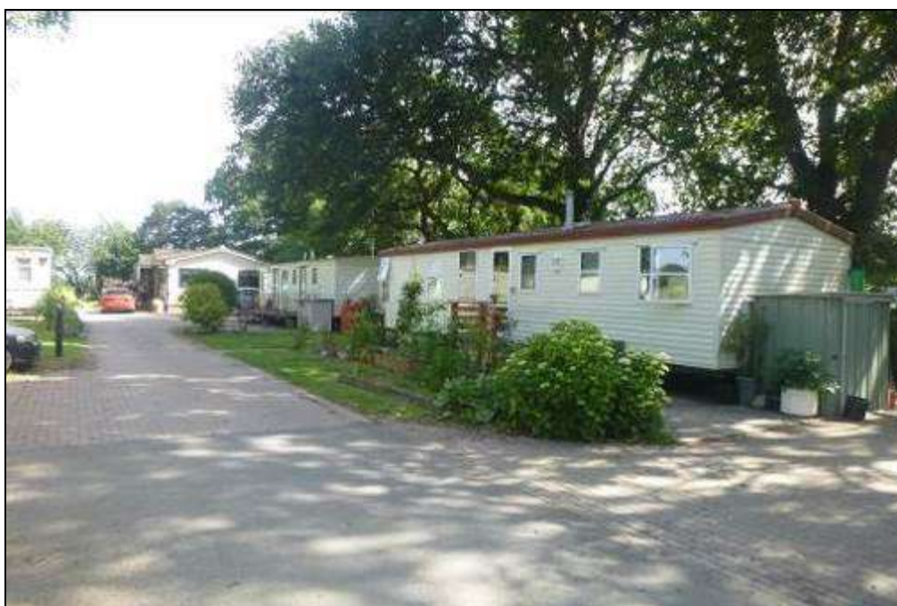
Photograph 8 Showing the mobile home park on the northern section
