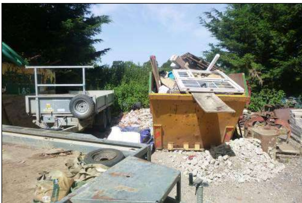
Photograph 6 Stored or discarded construction items to the north of the building
