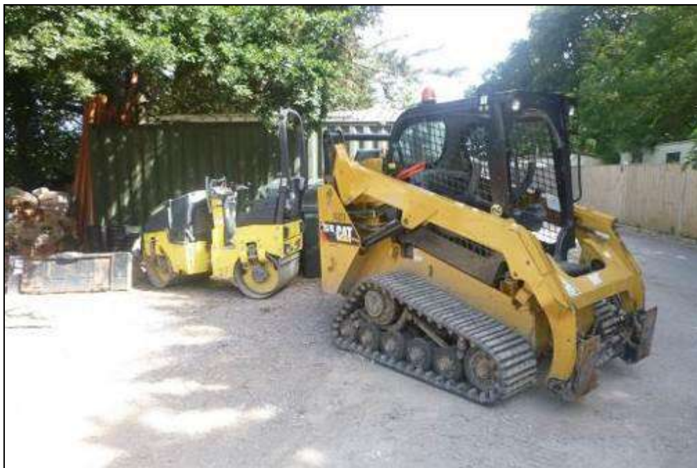
Photograph 5 Showing plant machinery to the north of the building
