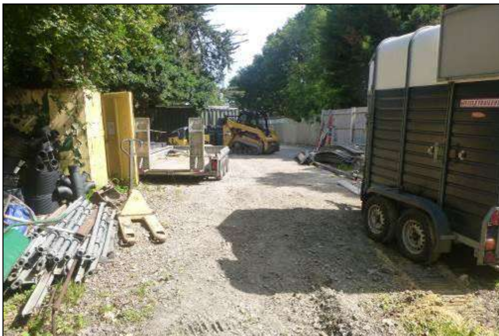
Photograph 3 Showing the area to the immediate north of the building
