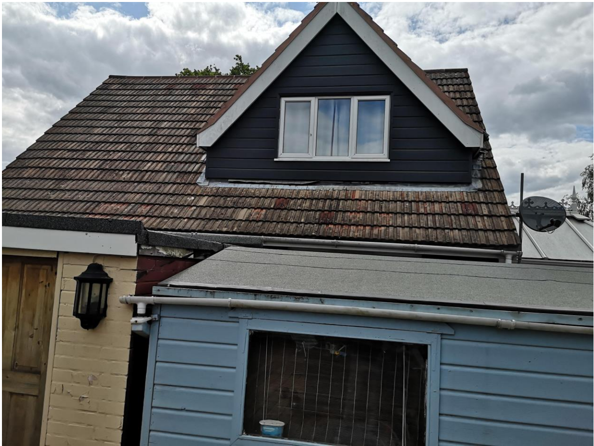
Photo 3: Side of No. 112
