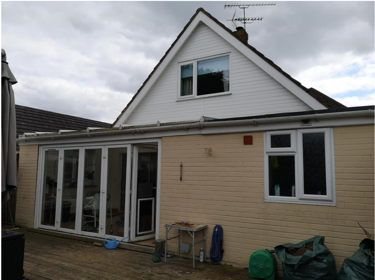
Photo 1: Rear of property
