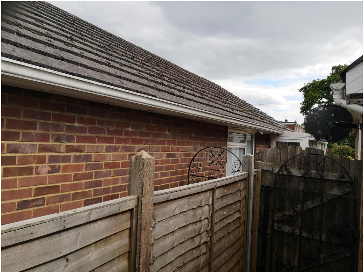
Photo 4: Side of No. 108
