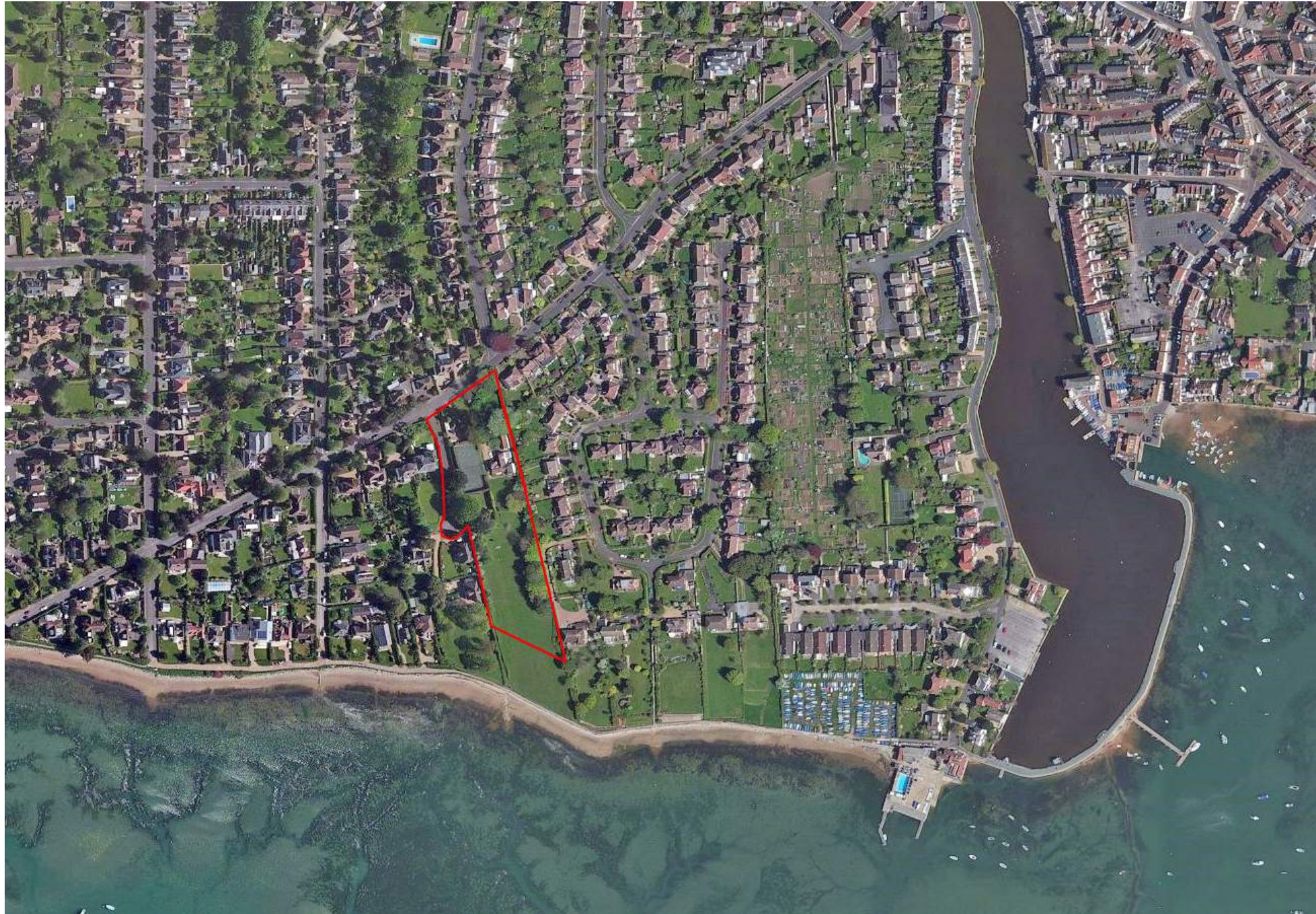
above Aerial view of site location
