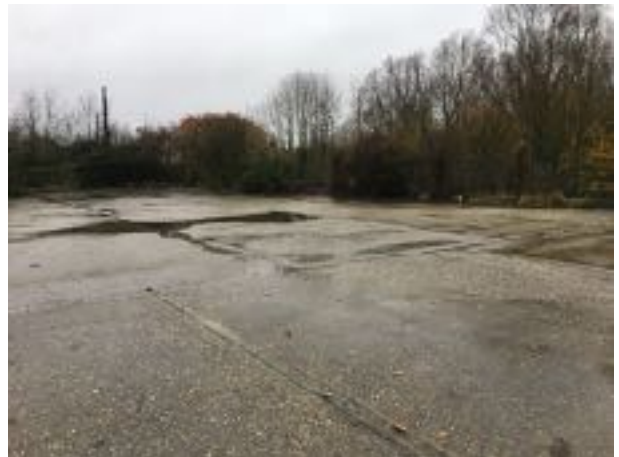
Figure 4 - Site looking northwest
