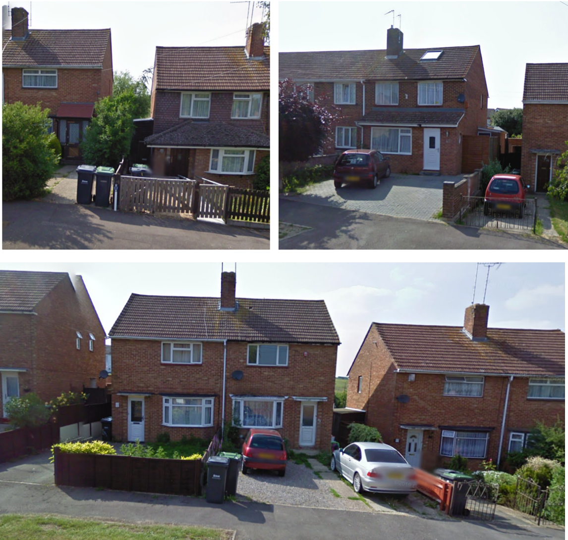
Figure 3 – Appearance of hard surfaced frontages on Winterslow Drive
