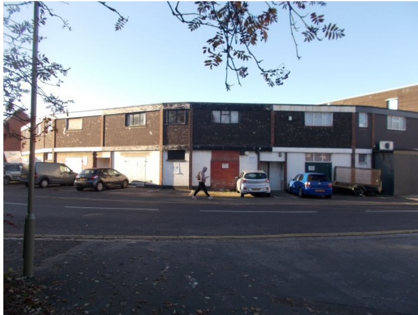
Fig 1. View of site taken from Prince George Street car park looking south.
