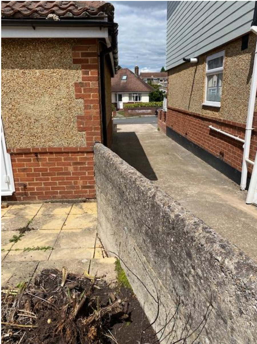
Photo 6: Side of the property
