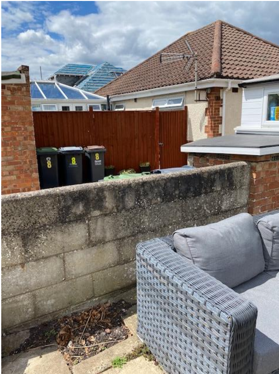
Photo 8: Side facing No.8 Alameda Way
