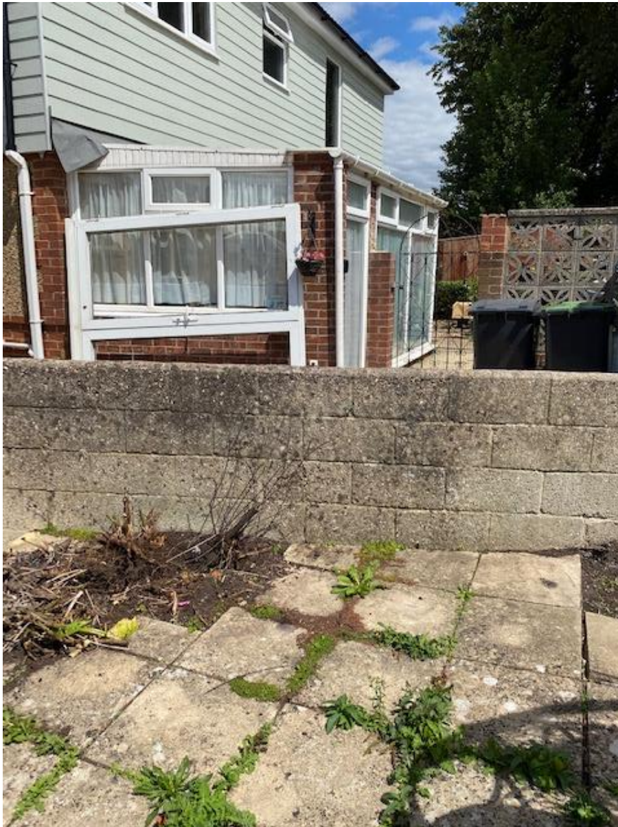
Photo 7: Side facing No.12 Alameda Way
