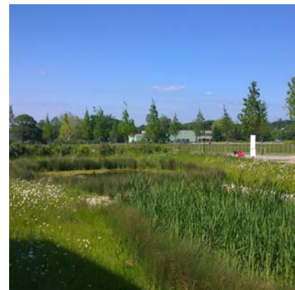
Example of SuDS basin
