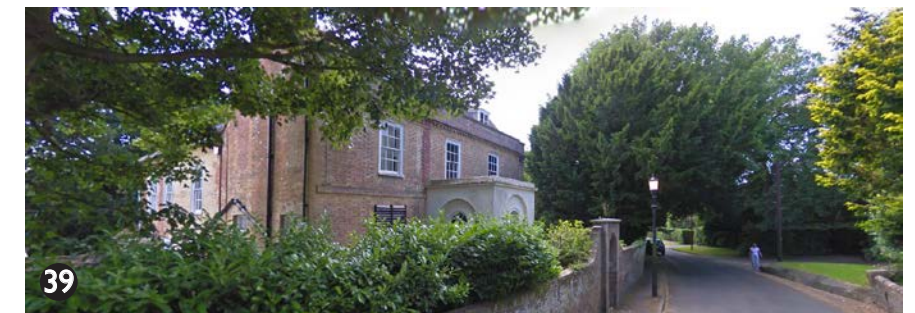
39 Old Rectory, Bidbury Lane, Bedhampton (Grade II listed, dates from late 18th century)
