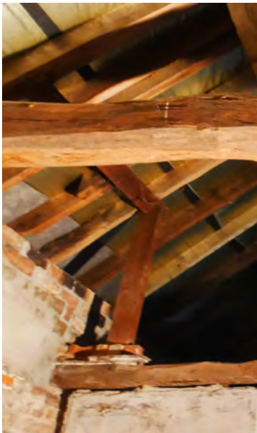
52. Later interventions to roof over wall between FF1 & FF12
