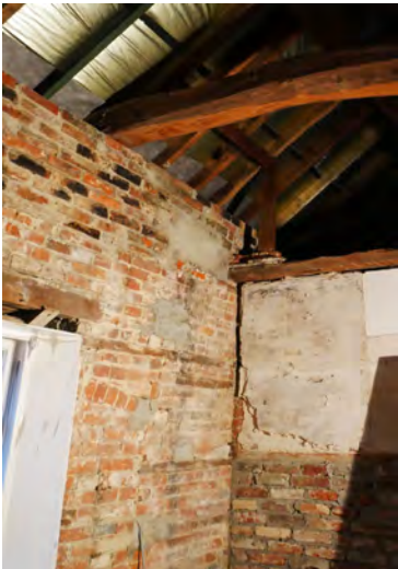
50. Similar view showing the blocked up door to FF12 and the cambered brick arch to former bay window. Again raised height evident.
