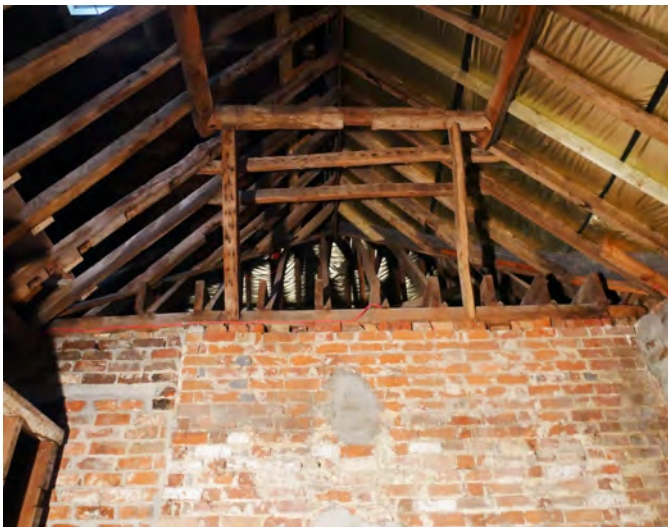
51. South inner elevation - wall plate to central chamber of 3-bay timber framed building noted with two extended areas of brickwork suggesting two phases of change and raised ceiling heights corresponding with raised floor heights to southern rooms. Note the nature of the Queen Post roof to FF5. Note the roof to the south differs over FF12 /13
