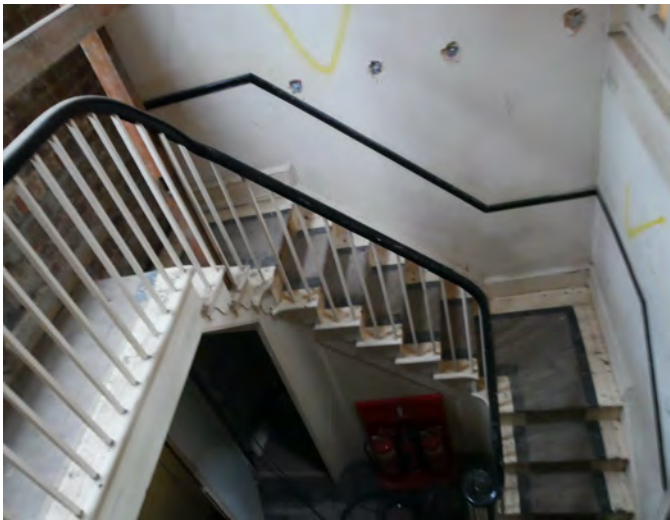
47. View of FF1 stairs and landings. The chair lift has been removed. Bolts noted through inner face of north wall. Note spindles are metal as the staircase has been altered.
