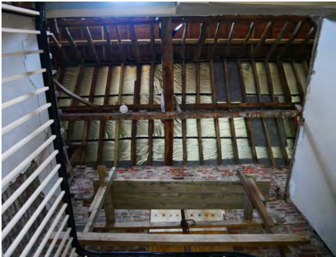
48. View up to underside of roof showing structure. The tie beam is pole stripped of bark, roughly shaped. The 'spine' is quite is lightweight and at the height of the former ceiling.
