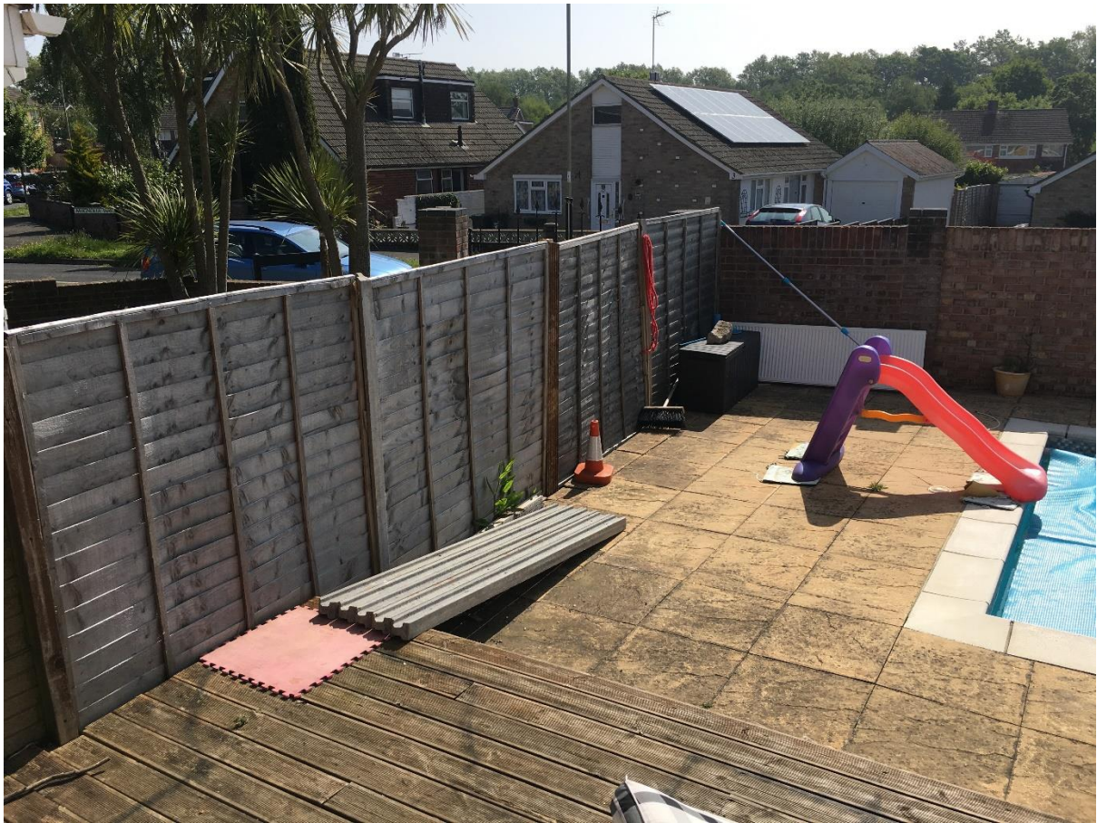
Photo 2: View from side Patio Door looking to the front
