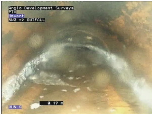
Photo: 6_6_29_A.JPG 0.2m, Water level, 50% of the vertical dimension
