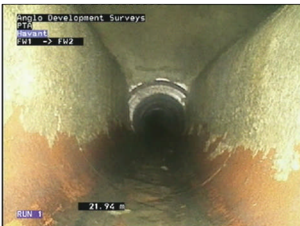
Photo: 1_1_8_A.JPG 21.9m, Finish node type, manhole reference number: FW2
