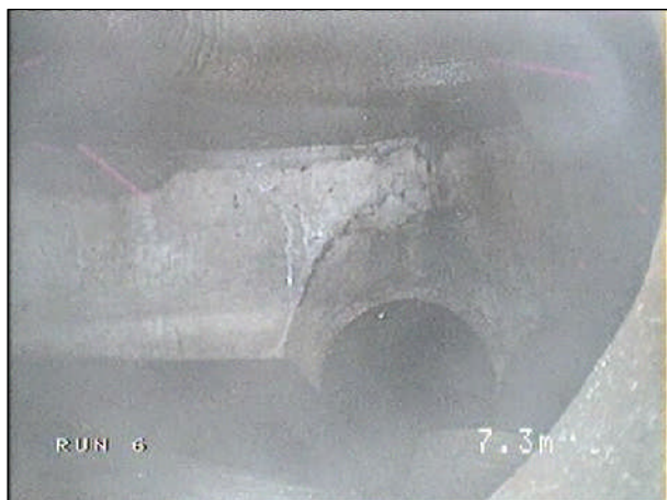
Photo: 7_7_41_A.JPG 7.3m, Finish node type, manhole reference number: OUTFALL
